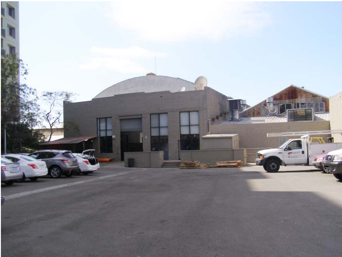
Photograph 2 - View of the rear of the building from the Valdez Street side
