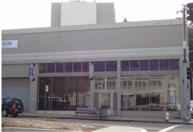
Photo 1: View of property (2800 Broadway), facing east.
