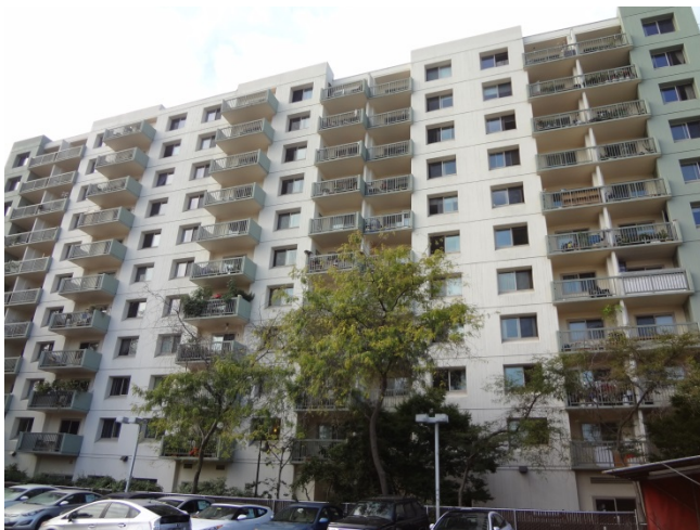
Photo 23: Southeast: Westlake Manor Apartments (262 28 th Street).
