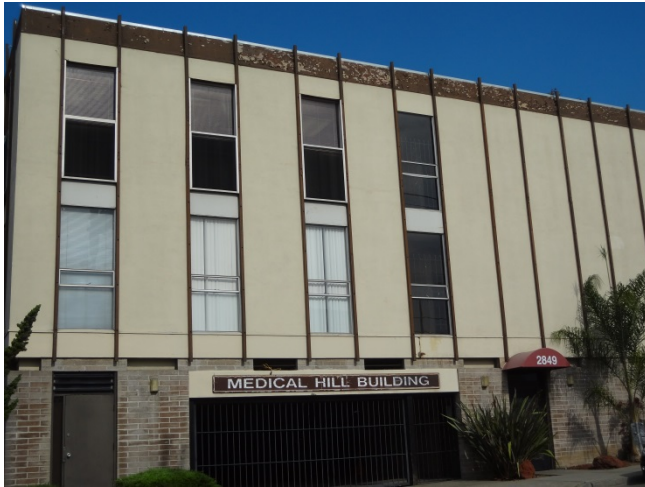
Photo 19: Northwest, beyond Webster Street: Medical Hill Building (2849 Webster Street)
