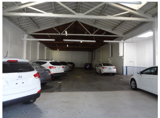
Photo 12: View of automobile storage at 2800 Broadway.
