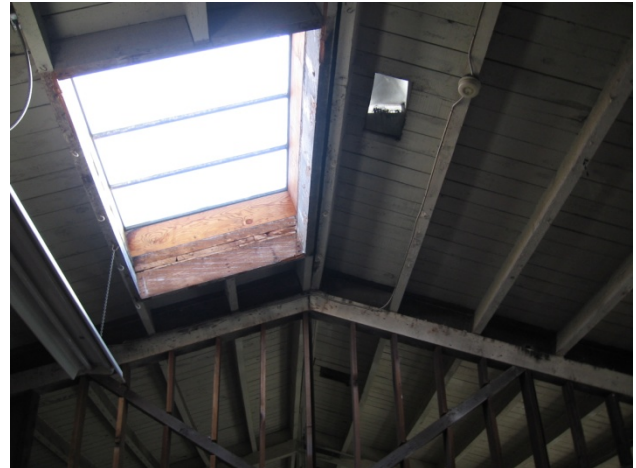
Photograph 10: Skylight in the upstairs office area.
