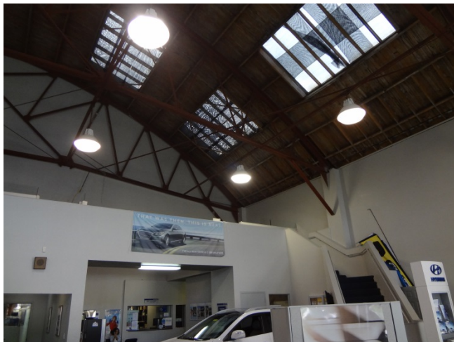
Photo 5: View of the mezzanine at 2820 Broadway.
