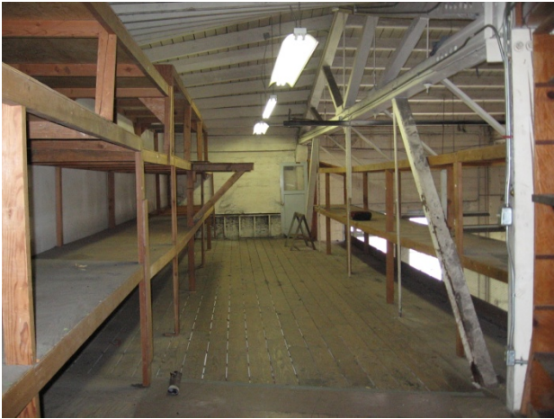
Photograph 7: The upstairs (mezzanine) area was formerly used for storage.
