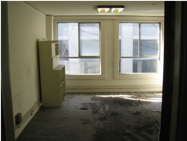
Photograph 9: One of the upstairs offices facing towards 28 th Street.
