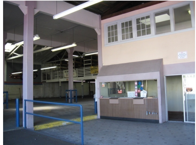
Photograph 4: The front showroom and the two-story office area. In the background is the mezzanine over the northern warehouse area.
