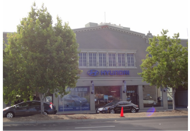
Photo 2: View of property (2820 Broadway), facing east.
