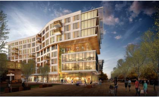
Jack London Square "F2", 338 du, under construction
