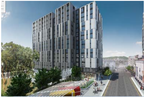
City Center "T5/6": 262 units, ground floor commercial, under construction
