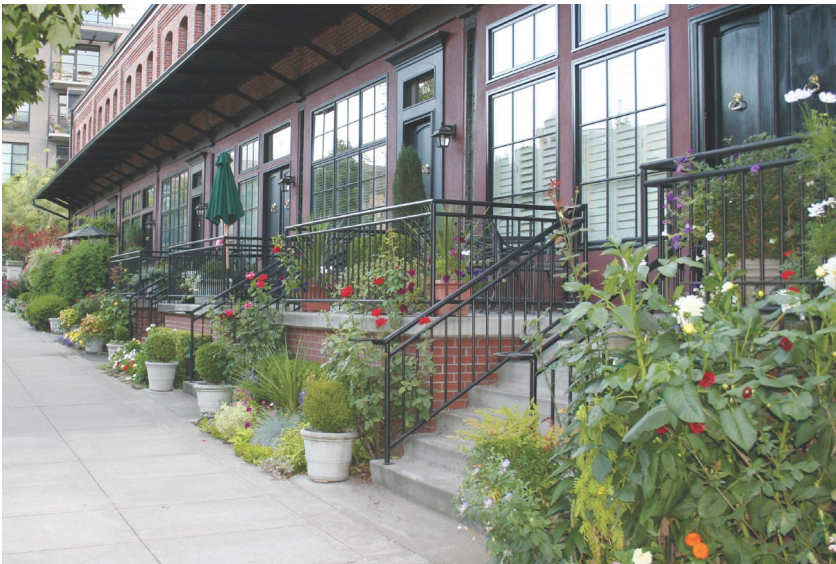
Patio or street front gardens are permitted along residential street frontages provided that they include landscaped garden walls and frequent entries. Individual unit entries with stoops are encouraged along street fronts.
