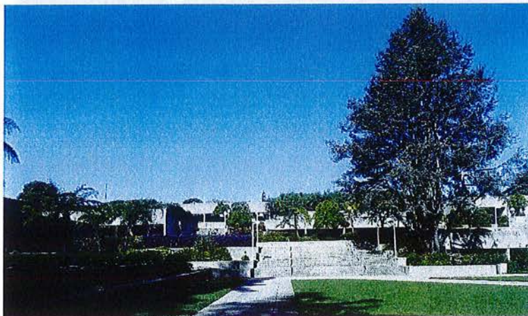
View of terraced building and landscaping, facing northwest.
