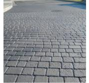
STAMPED ASPHALT PAVING
