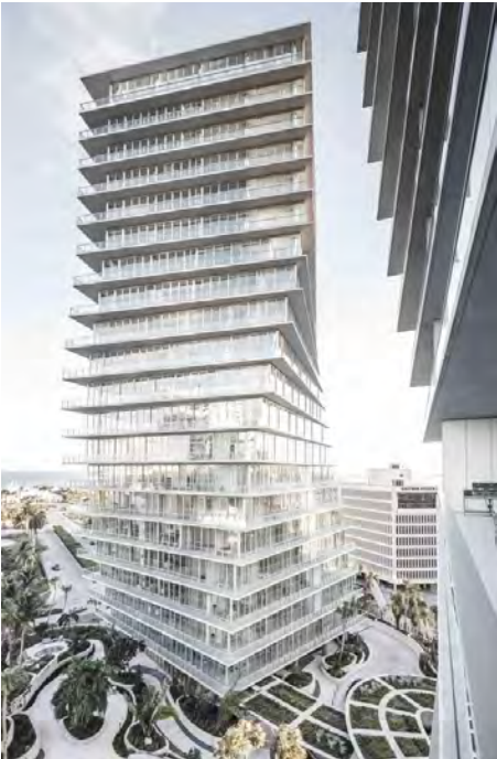
Figure 25: Shaping West Tower Facade
