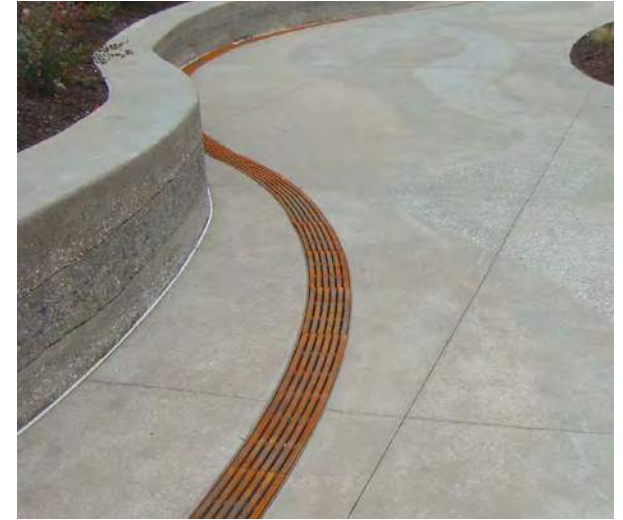
Figure 91: Trench Grate
