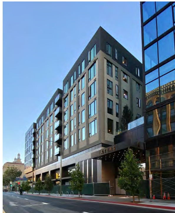
Figure 59: Mass Break between Buildings C and D
