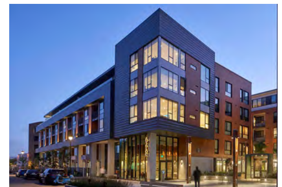
Figure 31: Building Corner at 8th and Fallon Streets
