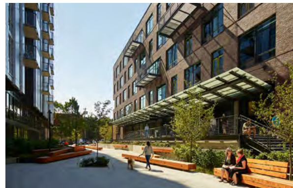
Figure 54: Community Room along Paseo
