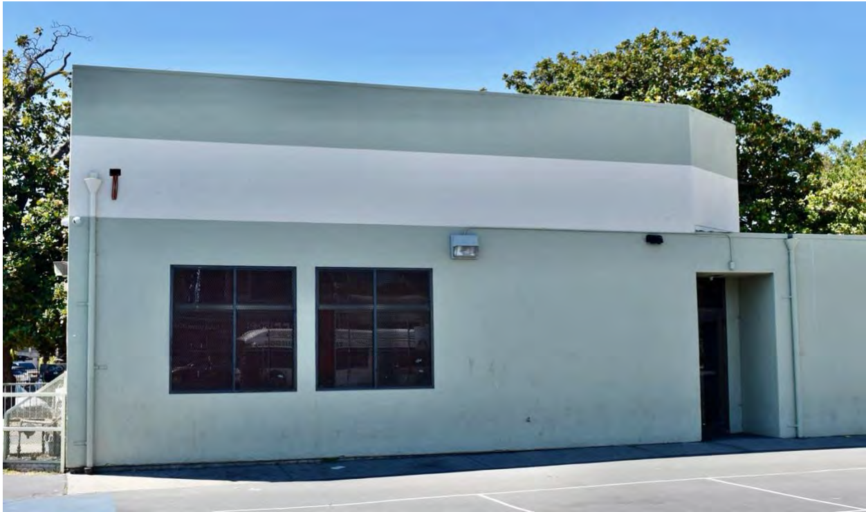
East wing, north façade
