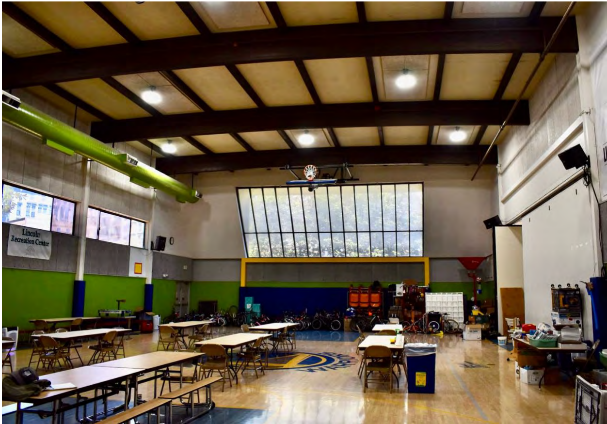
Multi-purpose room in west wing looking north
