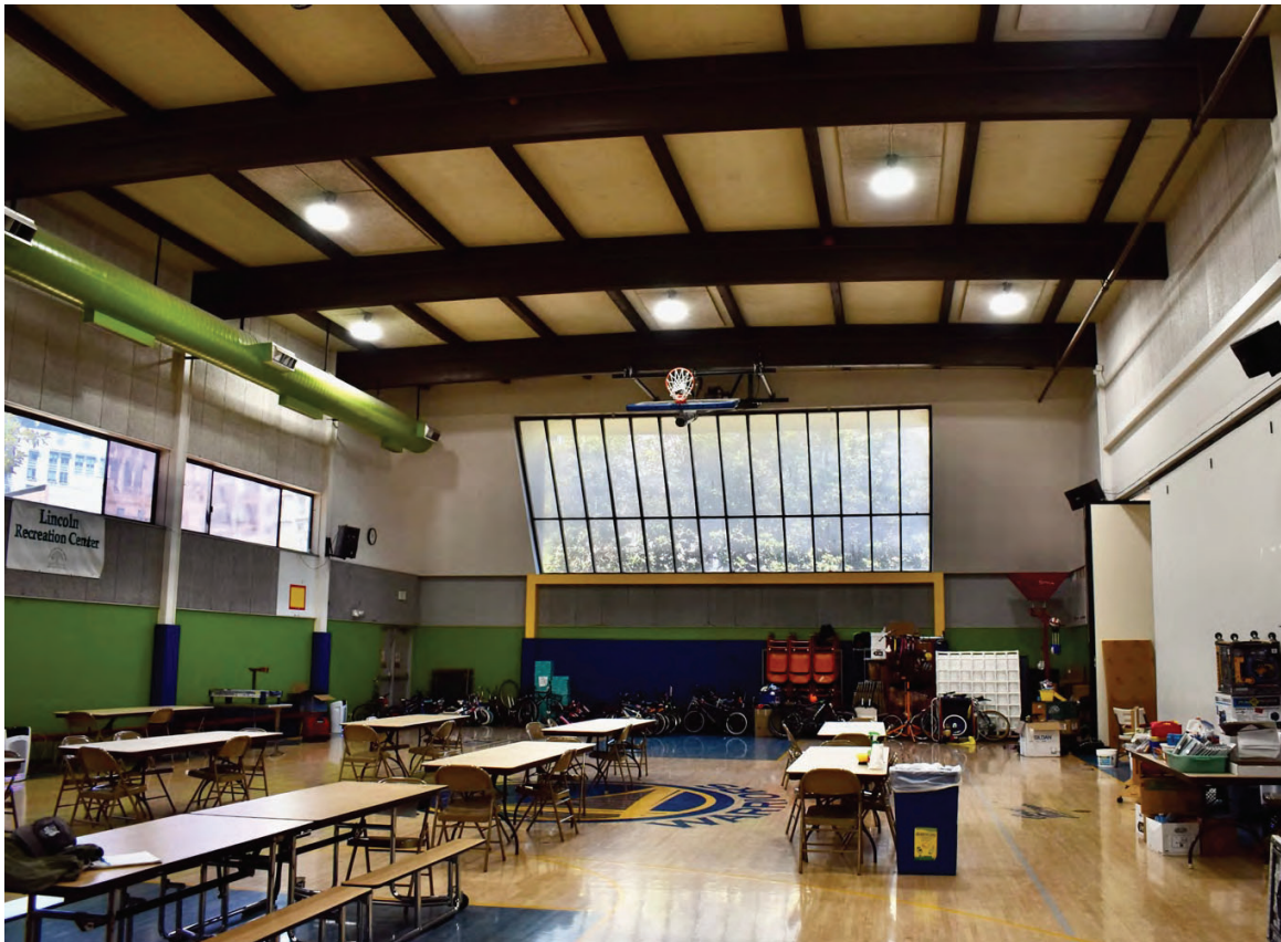
Photo 4: Existing Multi-Use Room in West Wing
