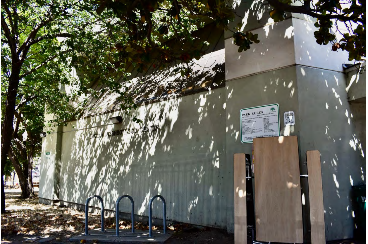
Figure 16: West wing, south façade from Tenth Street
