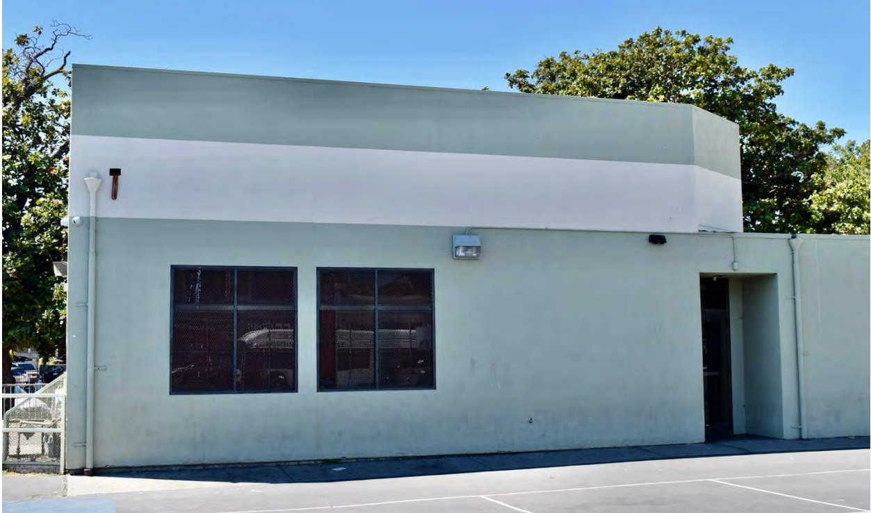
Figure 12: East wing, north façade
