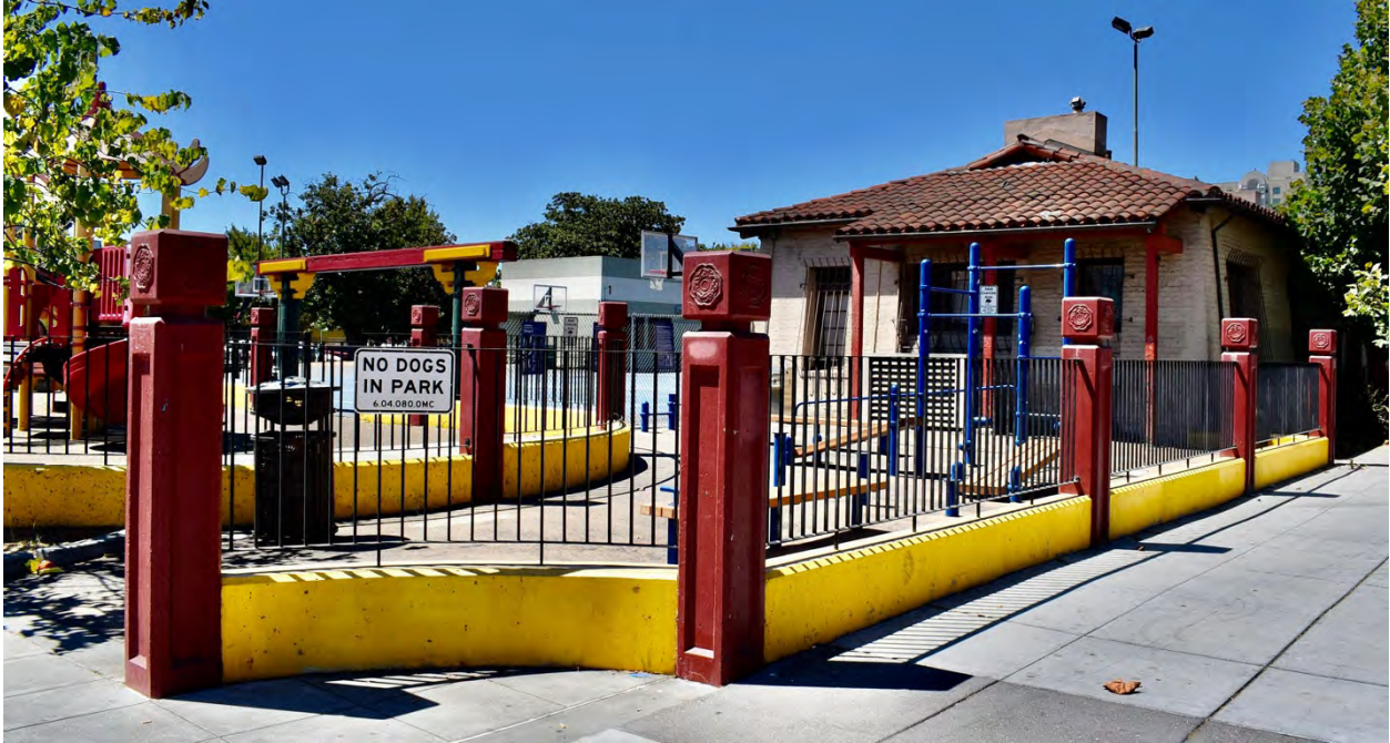
Figure 7: Park fence along 11th Street with Chinese style capitals, with Clubhouse at left
