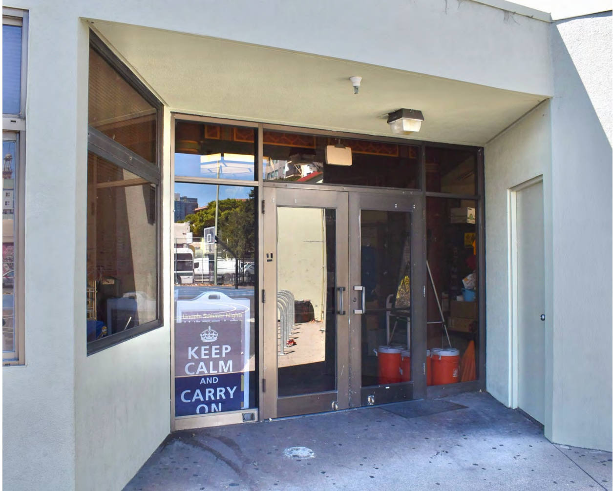
Figure 17: North entrance (from playground)
