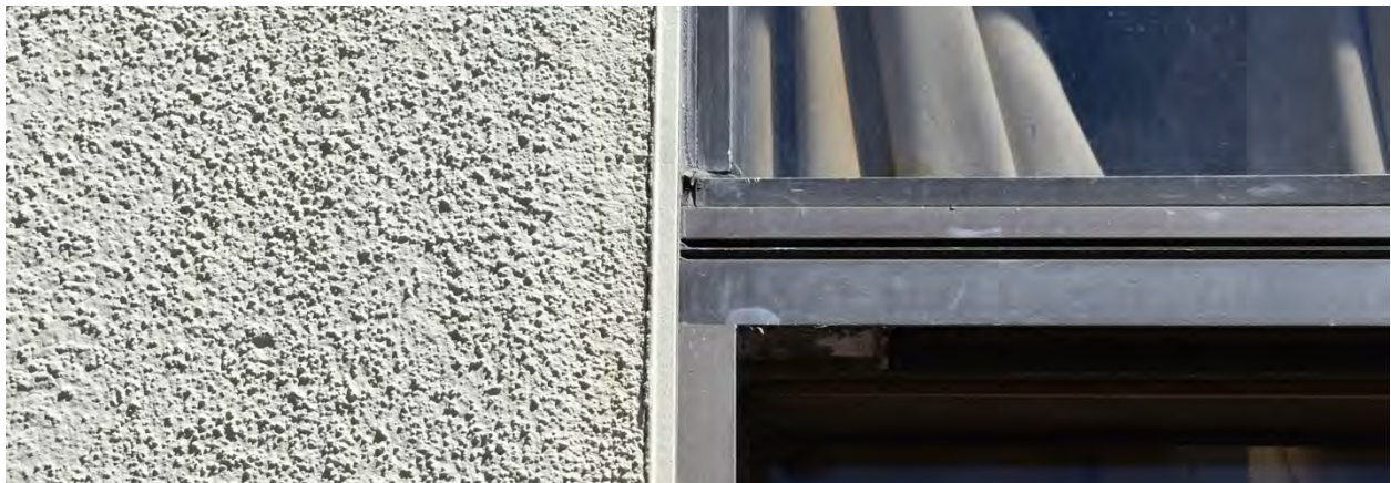
Figure 18: Window and stucco detail
