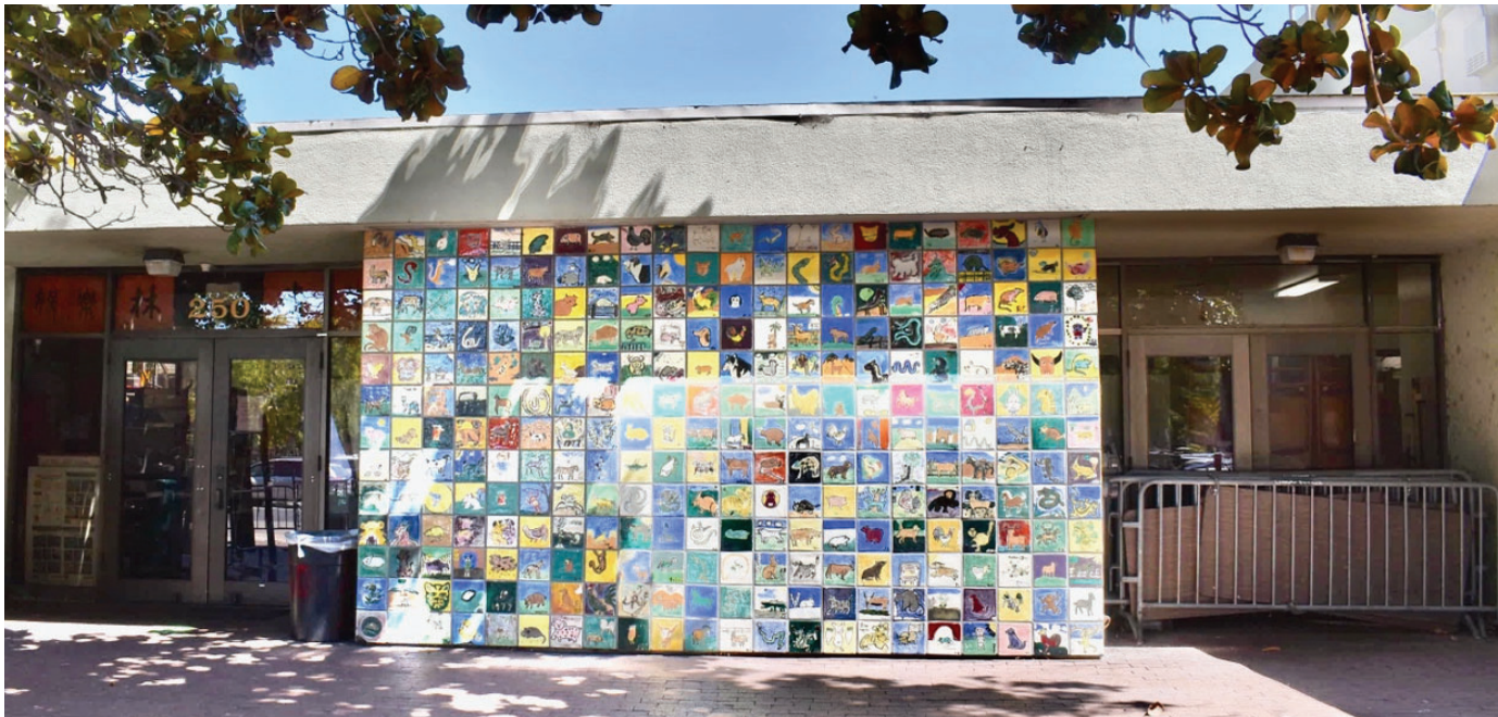
Photo 2: 10th Street Entrances With Tile Mural (South Façade)
