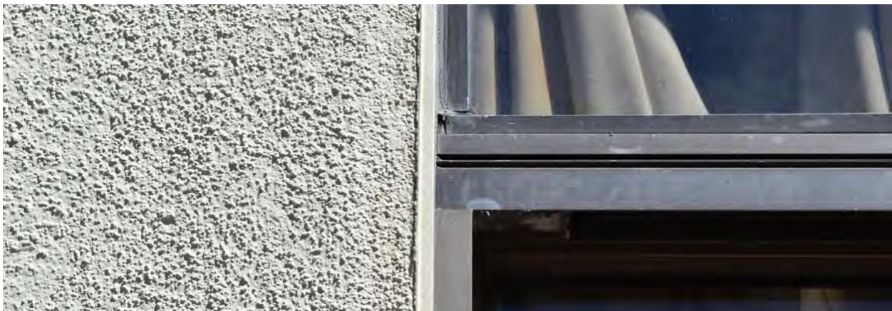
Window and stucco detail
