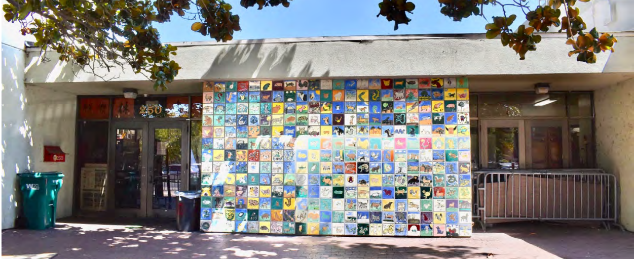
Figure 10: 10th Street entrances with tile mural (south façade)
