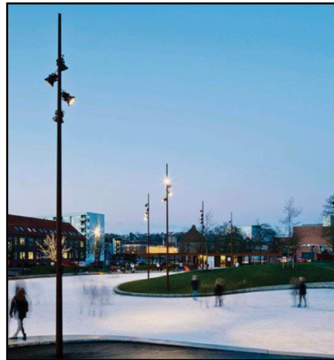
General lighting - Multi-headed pole
