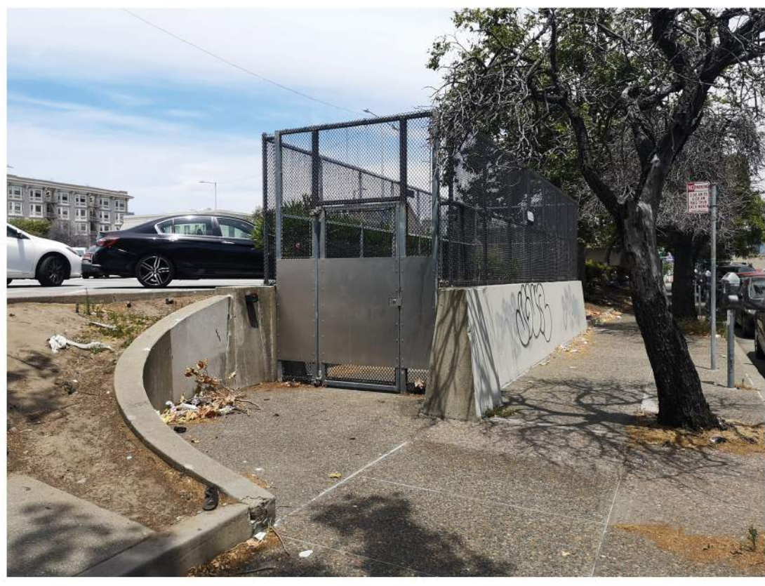
STAIR: TO REMAIN FINAL DESIGN TREATMENT TO BE DEVELOPED WITH BART. OPPORTUNITY FOR ART.
