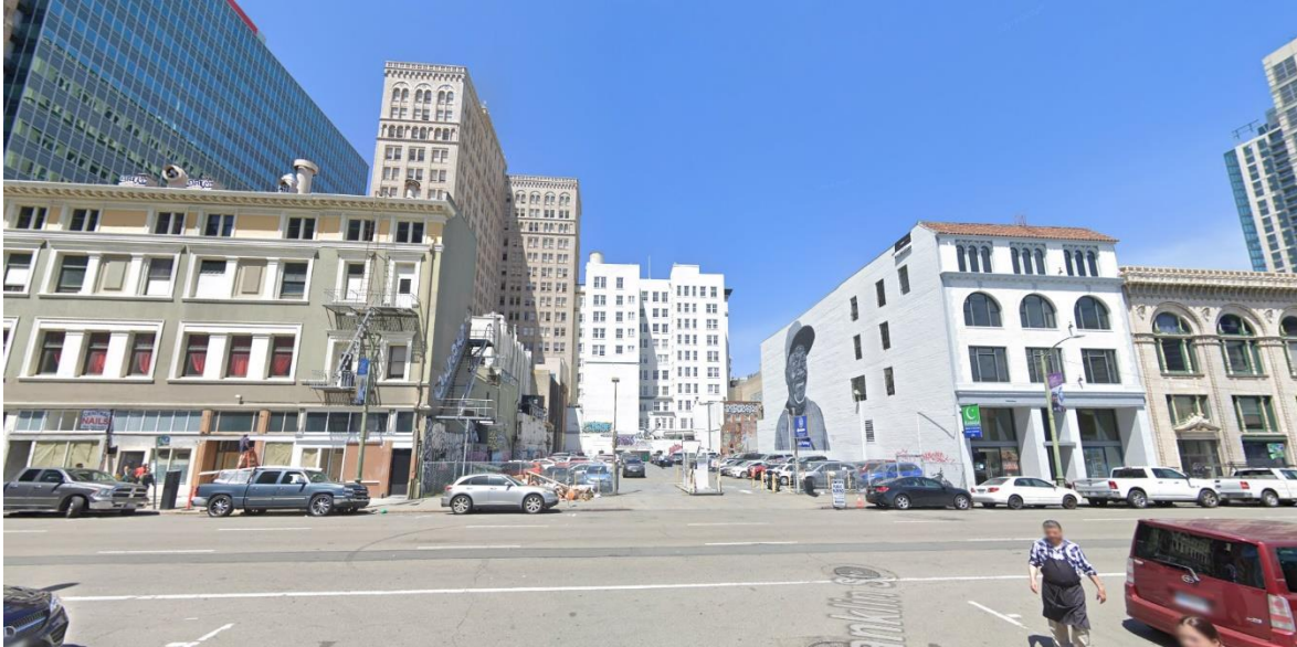
Photo of existing 1431 Franklin Street site.
