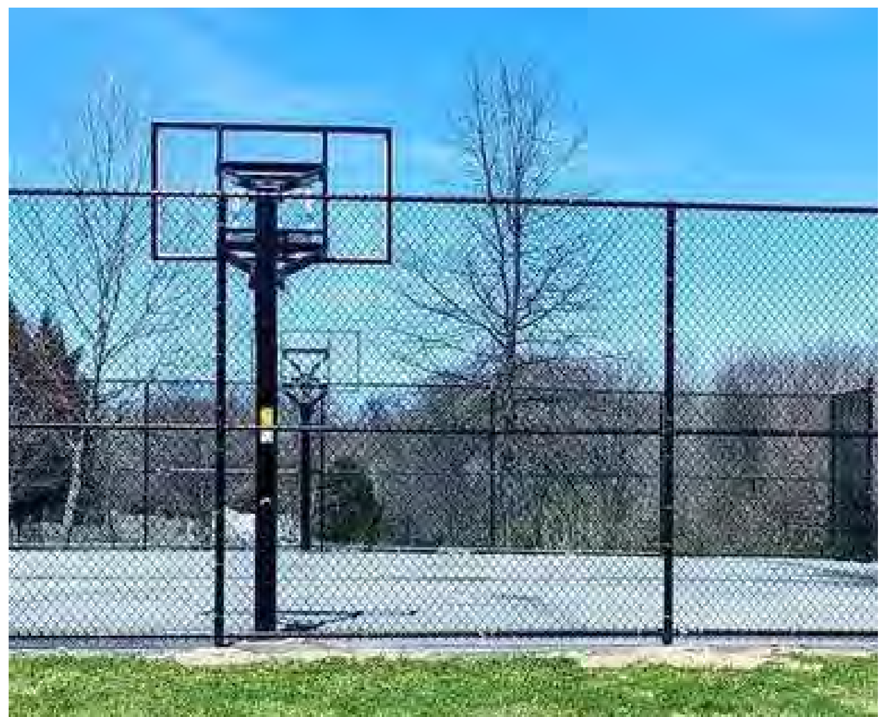
CHAIN LINK FENCE AT PERIMETER ADJACENT TO MULTI-USE COURT 10-FOOT TALL, BLACK VINYL COATED
