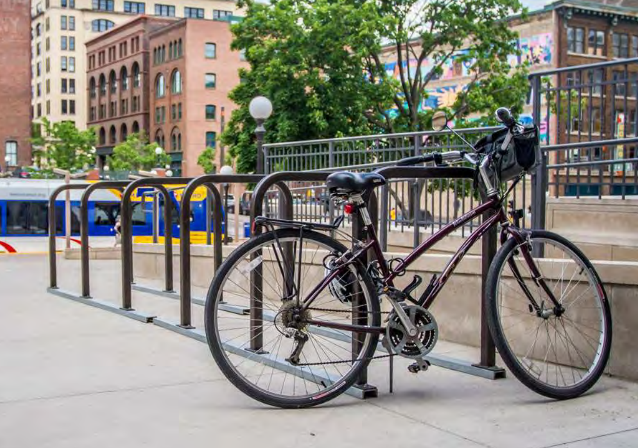
BIKE RACKS DOWNTOWN WITH CONNECTING RAILS FROM DERO COLOR: FLAT BLACK, RAILS ARE GALVANIZED
