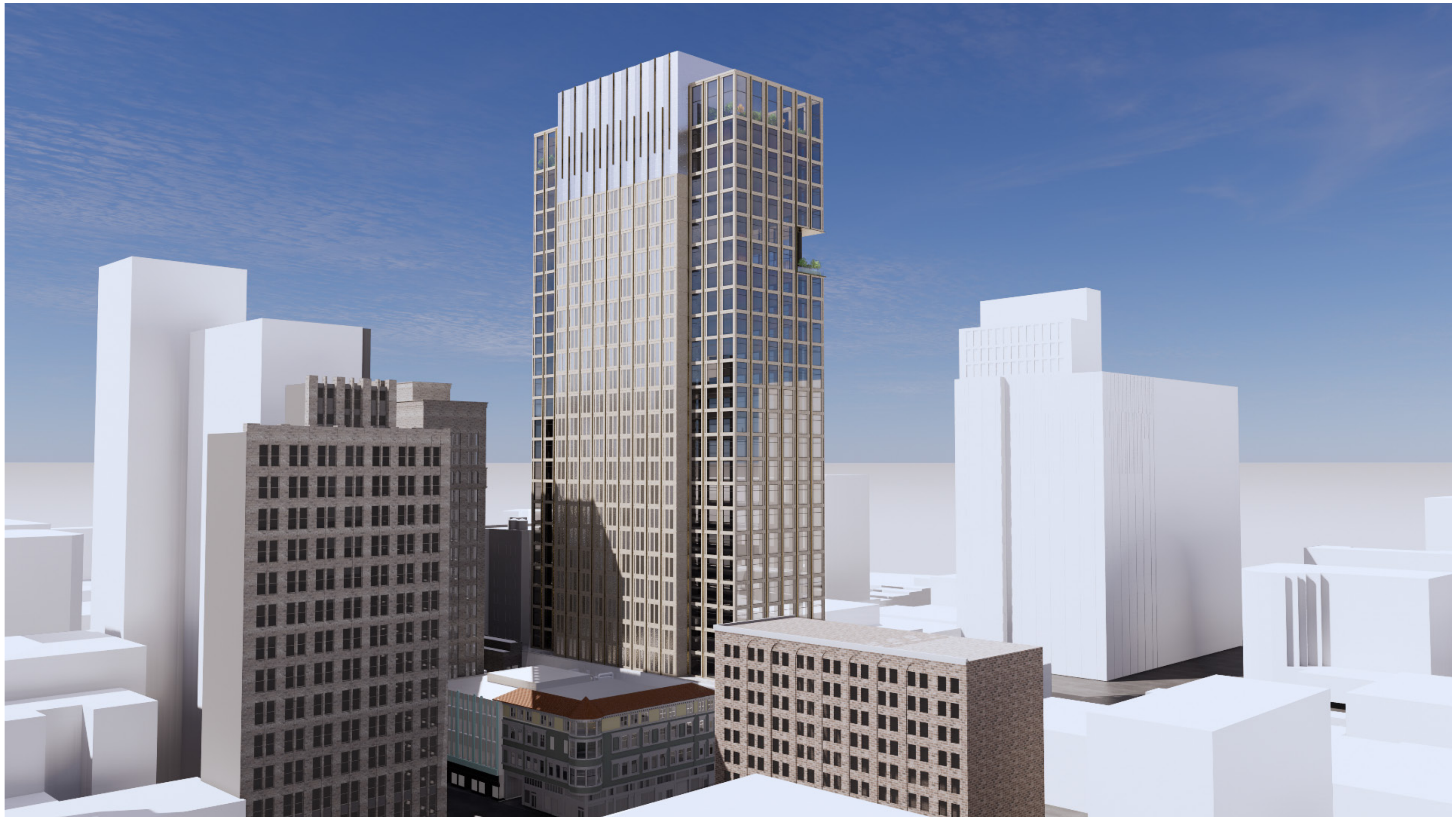
OVERALL LOOKING NORTH-WEST
