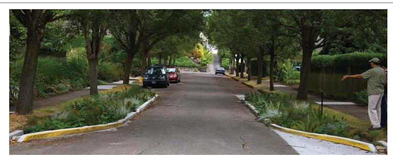
Typical Infiltration Bulb-out / Flow-through Planter / Rain Garden
