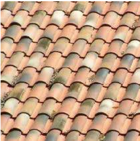
CLAY TILE ROOF
