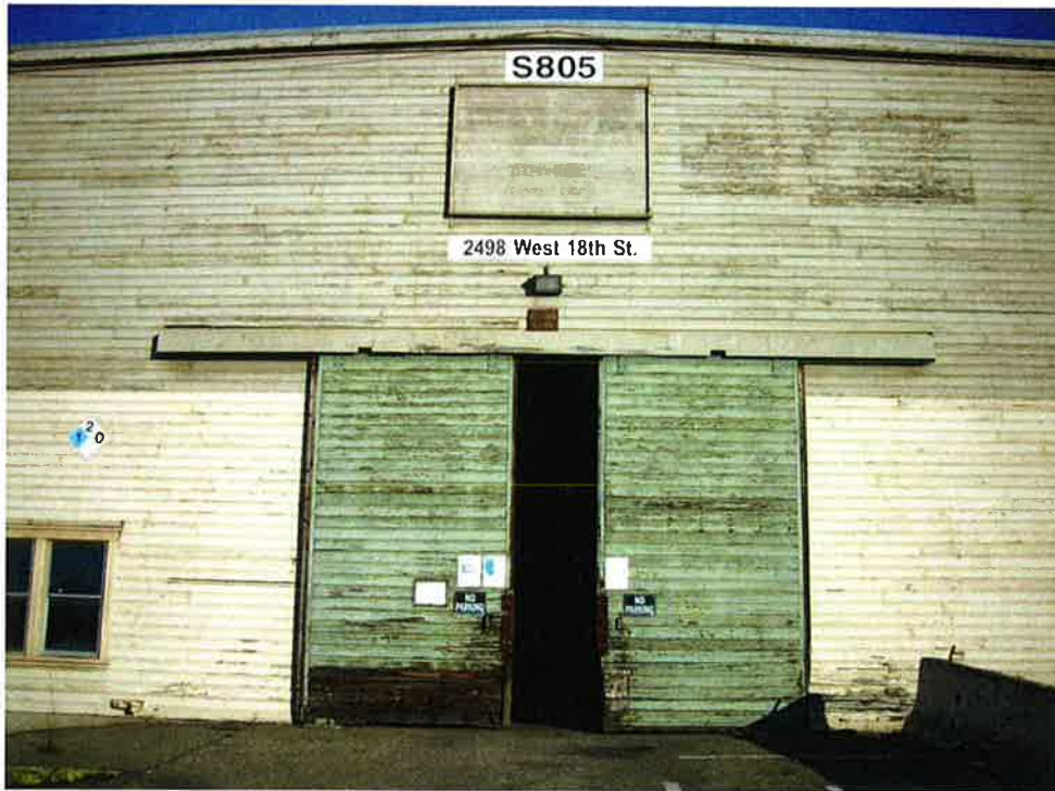
Photo 13: Weathered Siding
