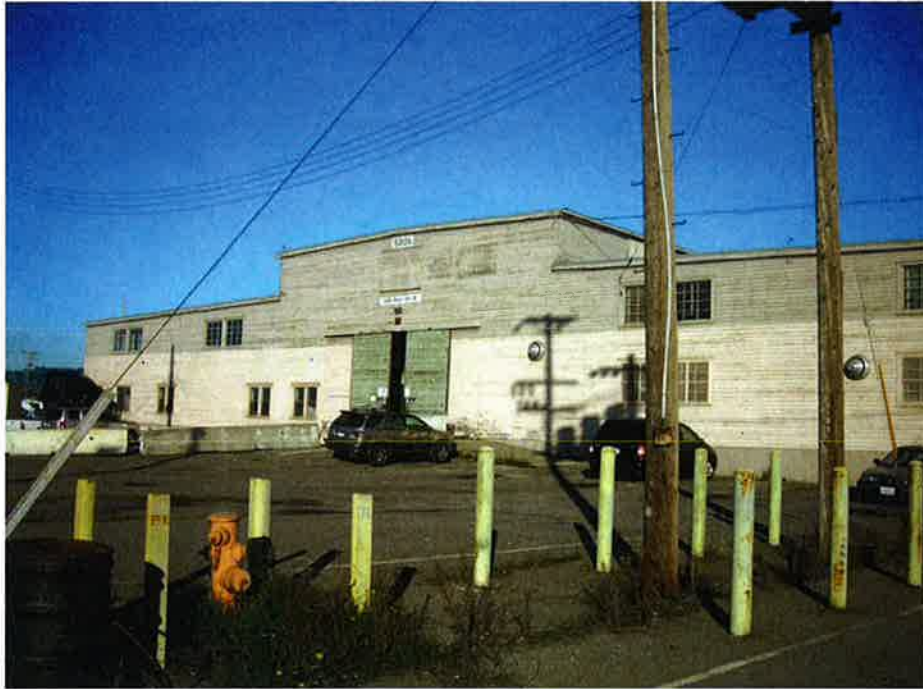
Photo 1: End Wall Elevation (West Wall)
