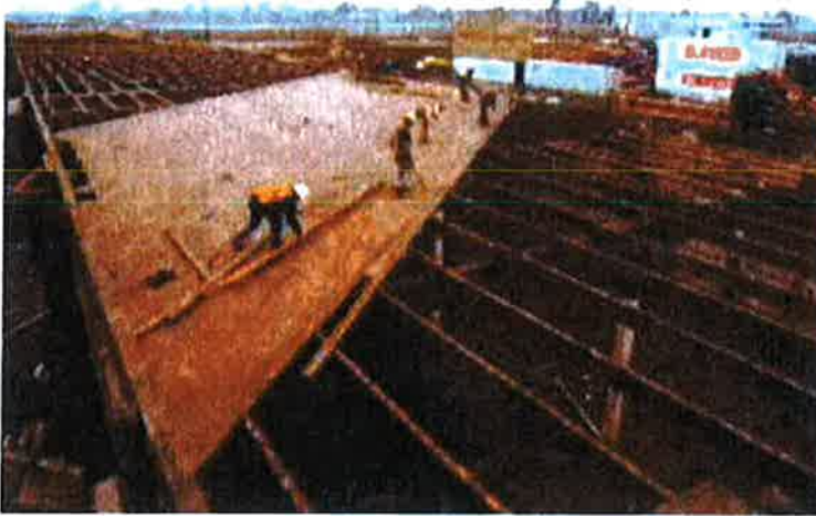
Figure 5.1- Roof sheathing removal
