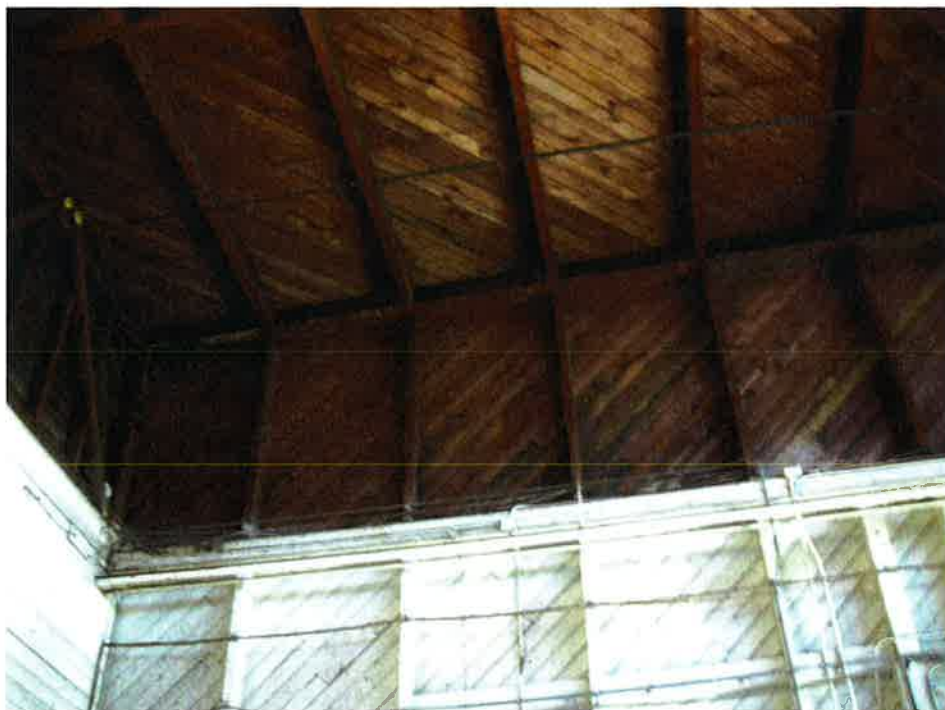
Photo 5: Wall/Roof Sheathing
