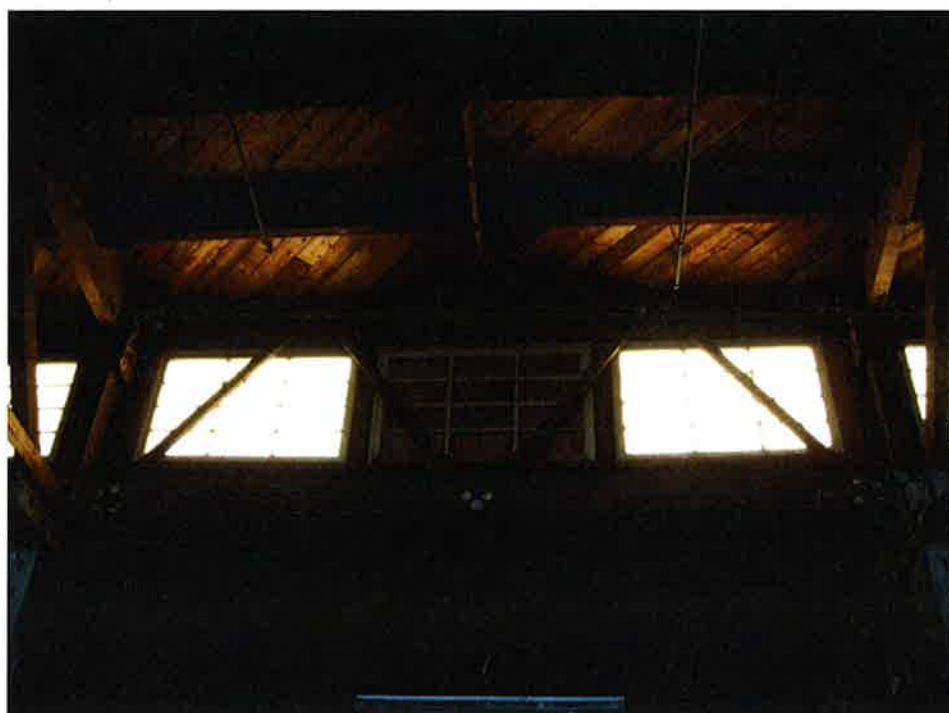
Photo 6: Clearstory Bracing
