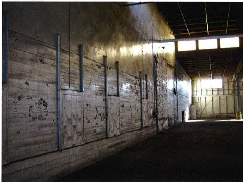
Photo 8: Typical Interior Partition Wall
