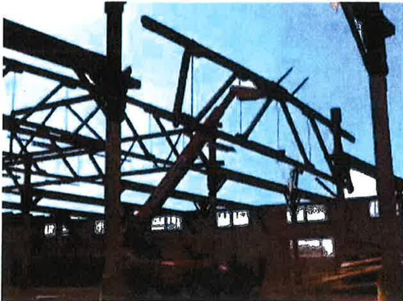
Figure 5.7 Truss removal
