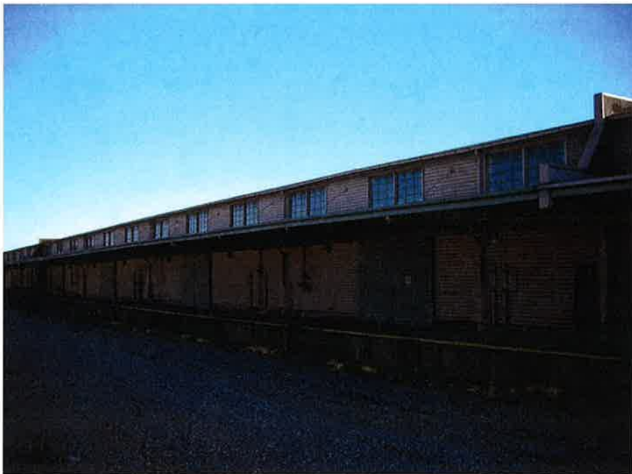
Photo 2: Side Wall Elevation (South Wall)
