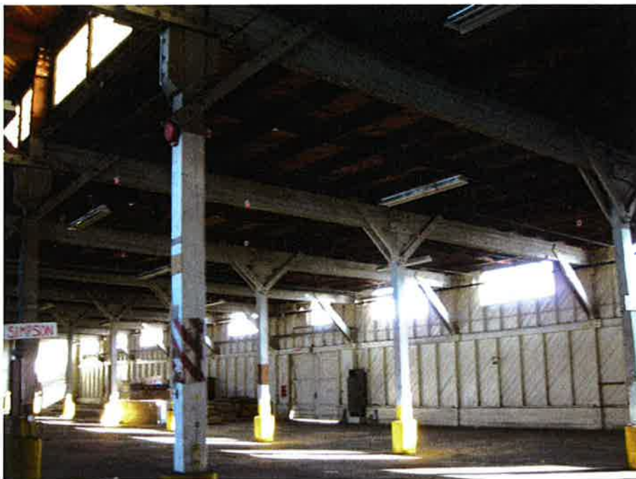
Photo 4: Framing at Low Roof
