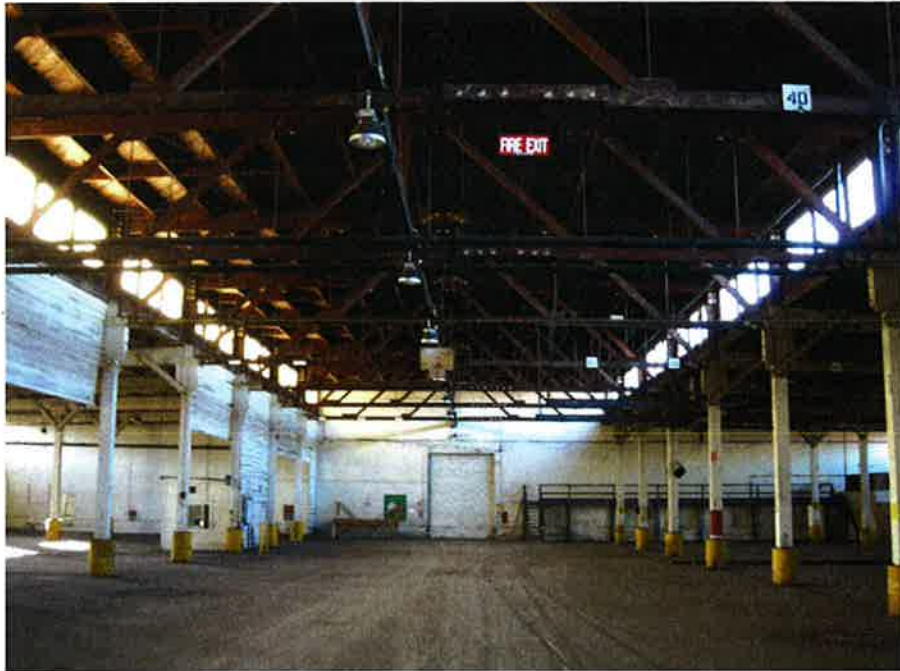
Photo 3: Roof Truss at Clearstory
