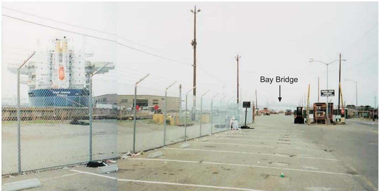
Typical views of industrial marine terminal facilities on the Outer Harbor.
