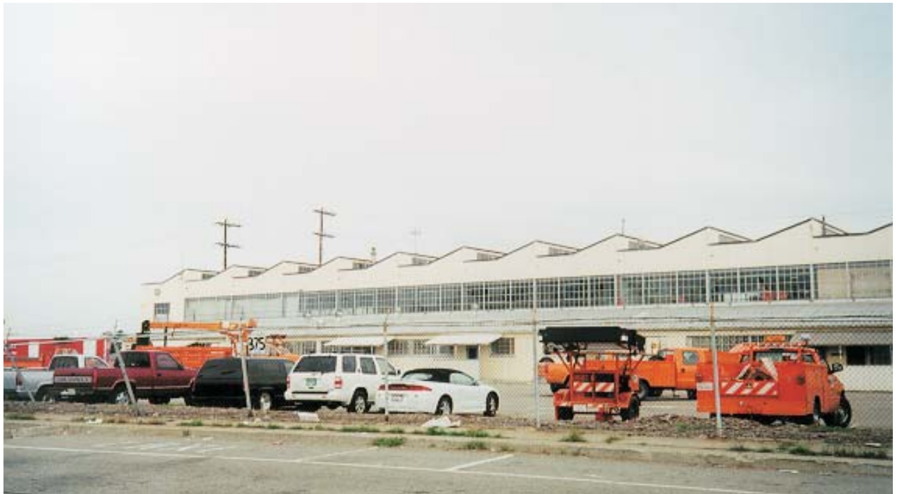
From Burma Road, view northwest toward Caltrans Bay Bridge touchdown maintenance facility.
