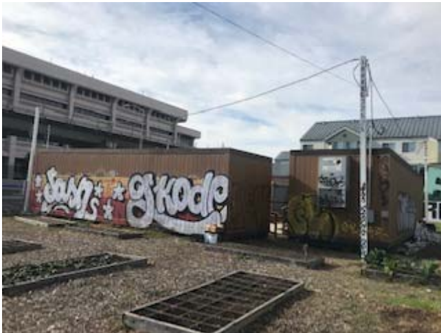
Photo 3: View of Portable Buildings on Target Property
