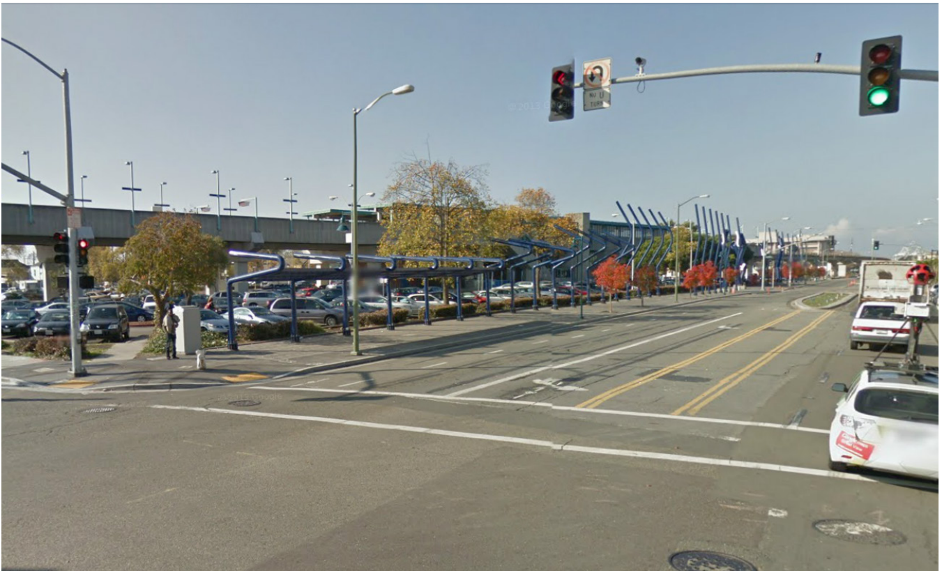
Fig. A-12: Existing view of West Oakland BART station at 7th Street and Mandela Parkway
