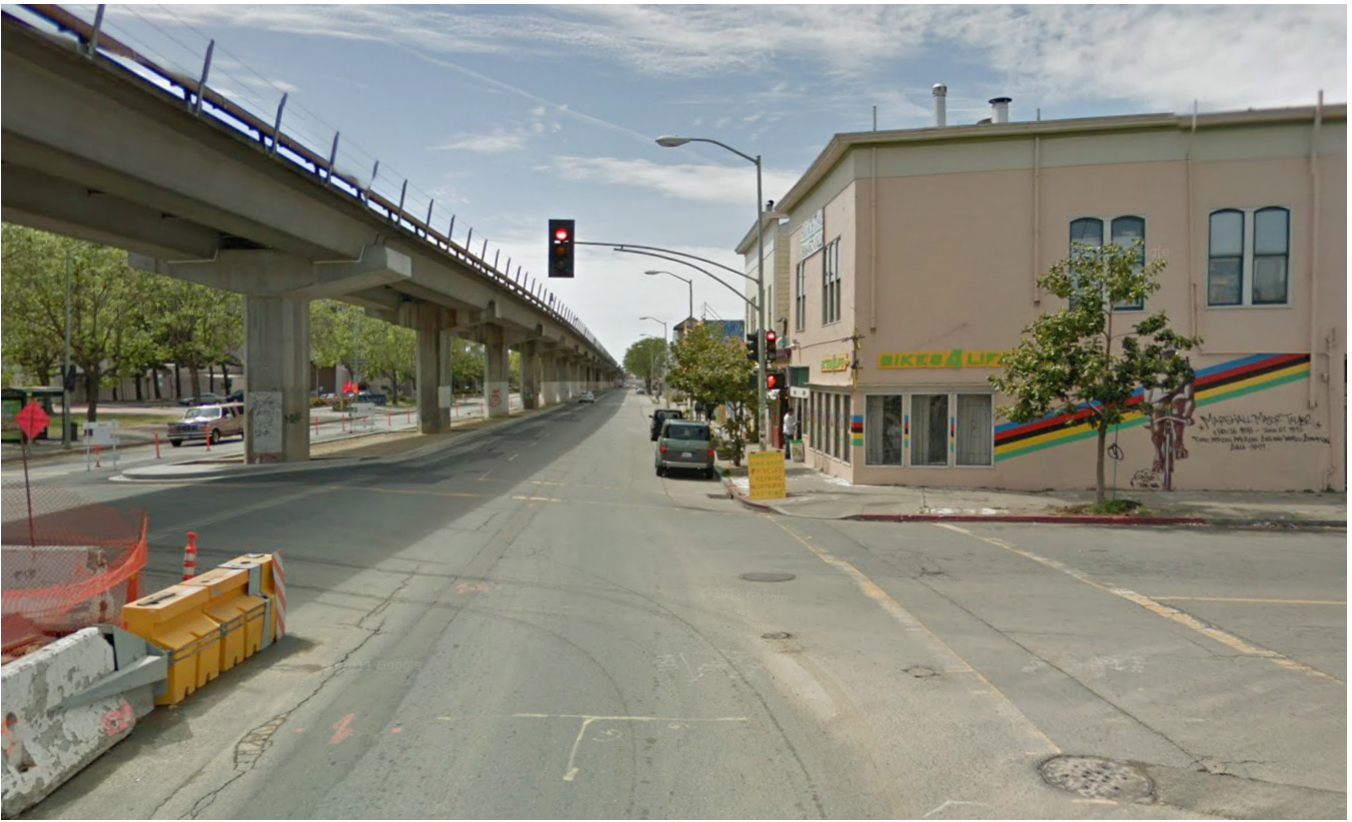
Fig. A-6: Existing view of 7th Street and Peralta
