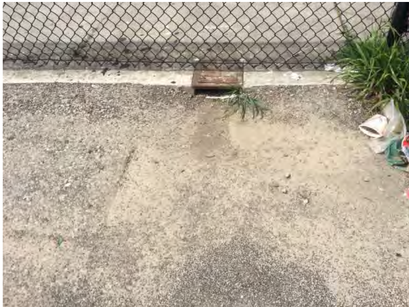
Subject Property Drain; Facing West
