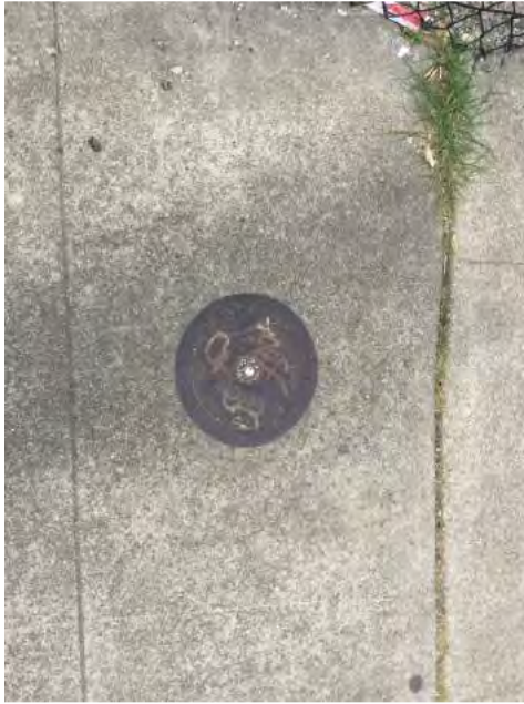
Former UST Fill Port; Facing North
