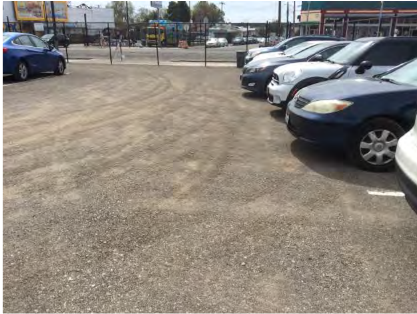
Subject Property Parking Lot; Facing South
