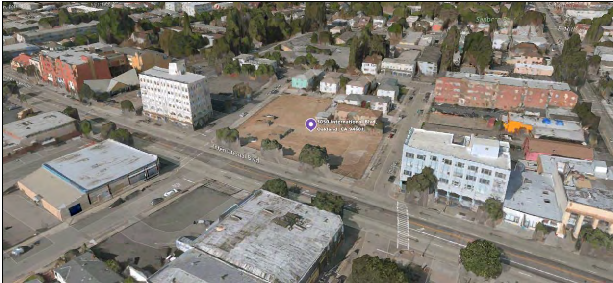
Figure 8 Aerial View/Existing Conditions
