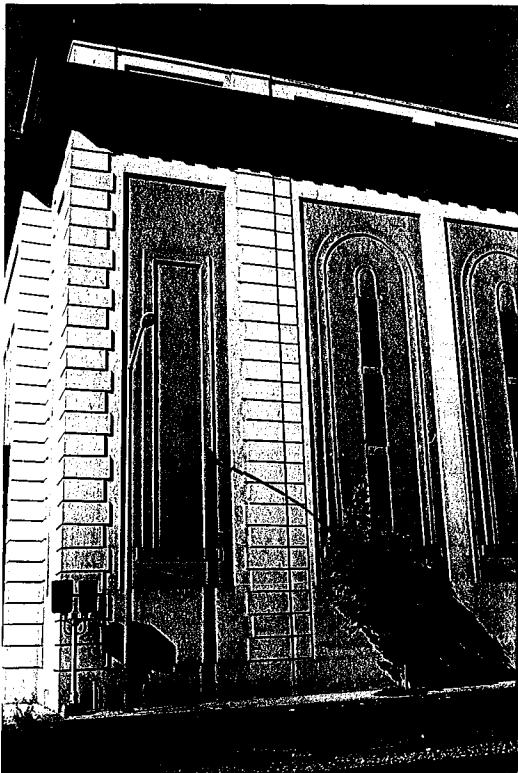
217-24 601 & 605 Embarcadero (P.G. & E. Station C) 5/82
