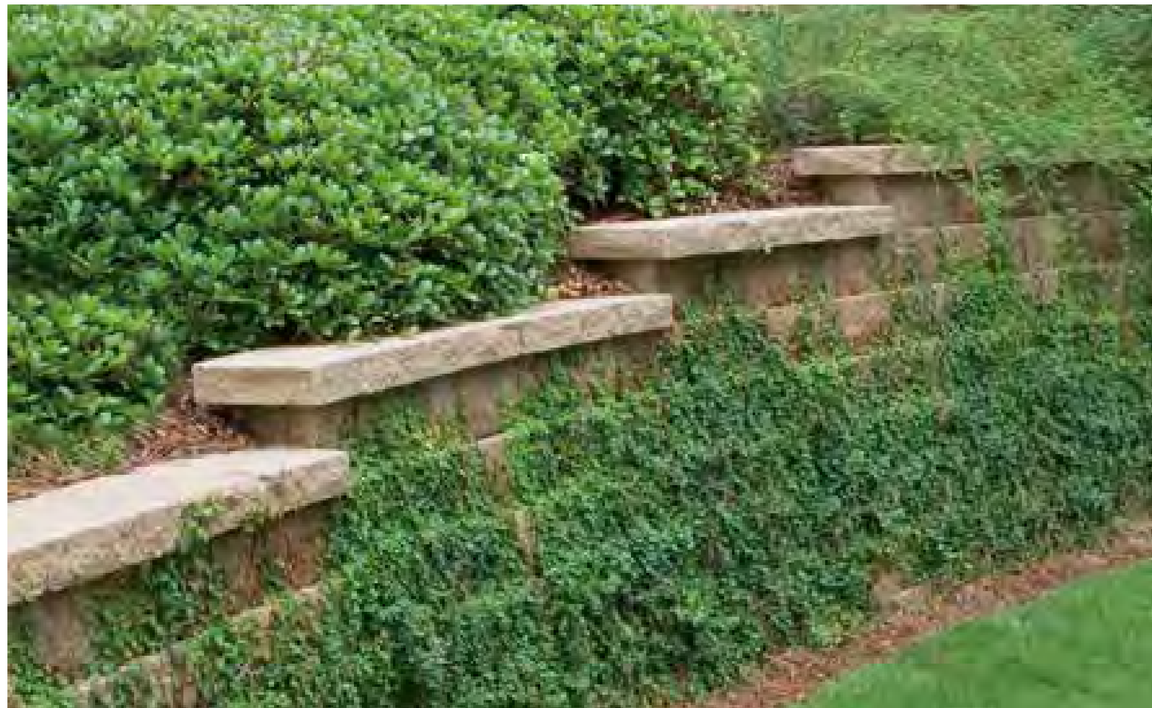
Pavestone 'Anchor Diamond Pro' retaining walls. Straight face style, Sandstone Blend color with vine plantings. Site walls shown on VTTM Sheets C.5.0 - C5.5.
