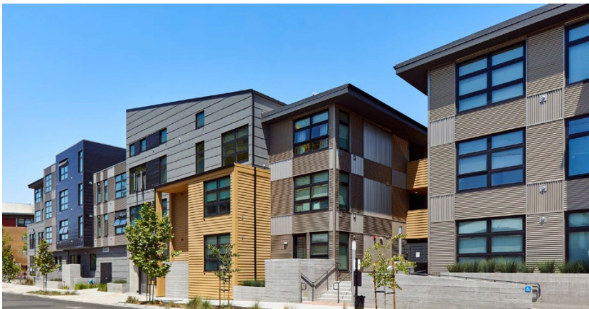
Recess and Projection in the building massing
