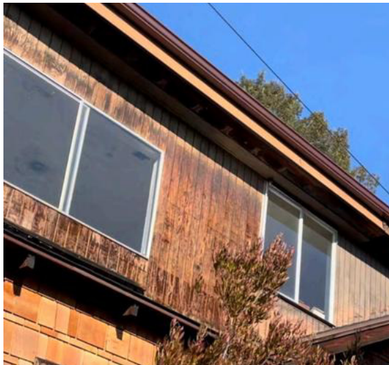
Left and Right: Replace 2 upstairs (S. and W. side) large aluminum windows Left: Replace 1 upstairs (S. side) alum. casement window with wood window
