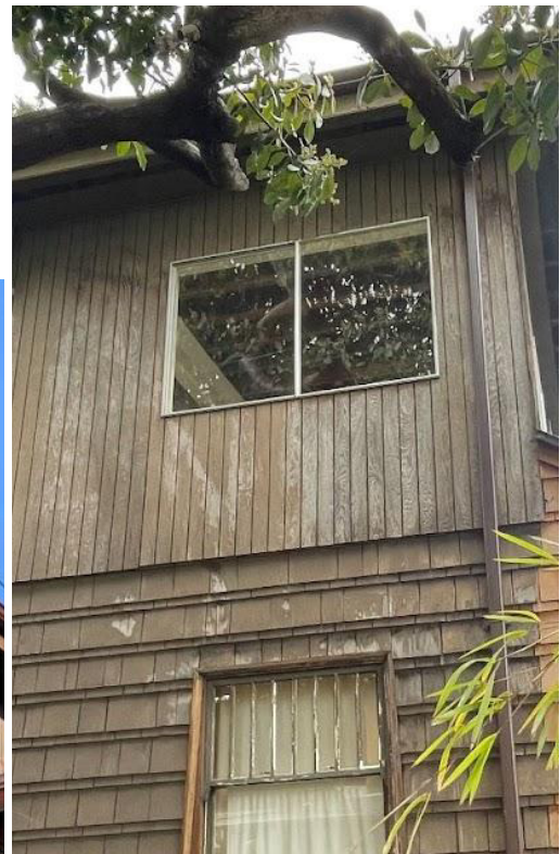
Left and Right: Replace 2 upstairs (S. and W. side) large aluminum windows Left: Replace 1 upstairs (S. side) alum. casement window with wood window
