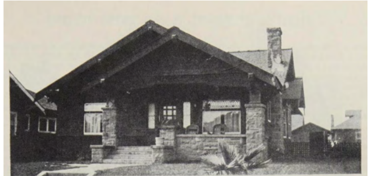
A SMALL CALIFORNIA BUNGALOW COSTING $3,200, SHOWING THE USE OF RED SANDSTONE FOR PORCH PILLARS, PORCH FOUNDATION AND CHIMNEY.
