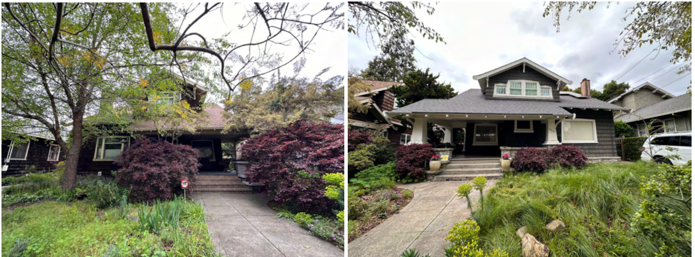
Houses at 5633 (left) and 5641 (right) Oak Grove Ave. Oakland CA
