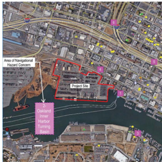
Figure 25: Receptor sites identified by ESA in their 1 February 2019 memo, indicating receptor site locations and numbers in pink. Note that the project boundary (in red) is incorrect; refer to the project boundary shown in the plan diagrams in Section 3 above.
