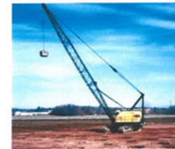
Figure 12.2.1. Example of deep dynamic compaction.
