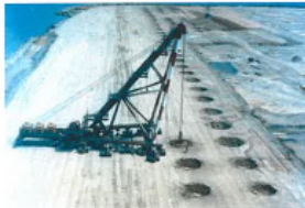
Figure 6.15. Menard's "Giga" compactor drops a 200-ton weight. Courtesy of Menard.
