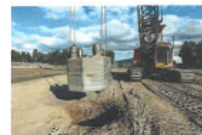
Fig. 2.6. Dynamic compaction. (A) Dropping of weight from a certain weight ( M_{max} ); (B) Drop locations.
