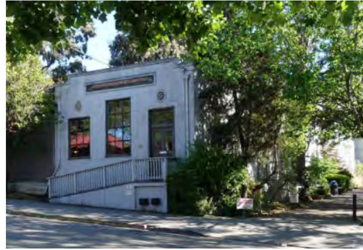
06 | Facilities Building on Clifton
