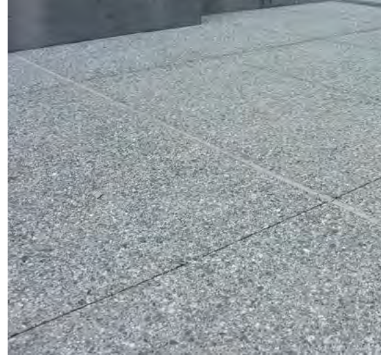
2. CIP Concrete Paving - Finish 2 Pedestrian and Vehicular
