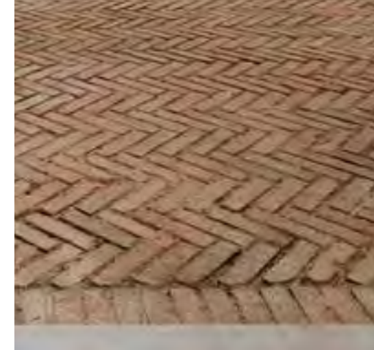
4. Site Salvaged Brick Paving
