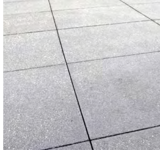
3. CIP Concrete Paving - Finish 3 Pedestrian
