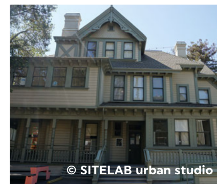
Figure 2.4: West porch (historical primary entrance) (above) and east porch to Macky Hall (below)
