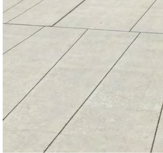
1. CIP Concrete Paving - Finish 1 Pedestrian and Vehicular
