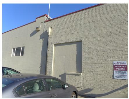
Original exterior brick walls and board-formed concrete wall of the south elevation (Carey & Co., 2015).
