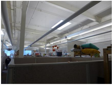
Timber columns and steel beams of the warehouse on Madison Street side (Carey & Co., 2015).
