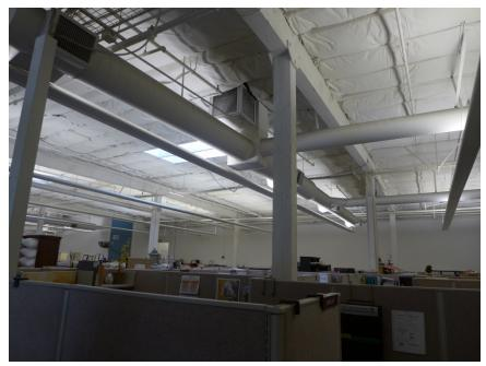
The painted heavy-timber columns and beams of the warehouse on the Jackson Street side, the roof is obscured by insulation (Carey & Co., 2015).
