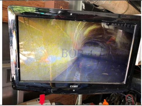
Work Item #1 - Photo 3 Robot "BOB-4" with camera. TV view of the poured concrete 100 plus year-old culvert directly under 901 Trestle Glen Rd (2019). Install three grade beams to further separate the house from the culvert 17-ft below the house grade level.
