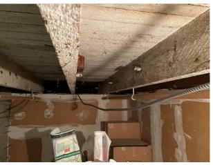
Observe the absence of shear transfer ties or blocking between joists.
