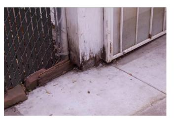
Observe this rotten door casing. All wood with ground contact will be repaired or replaced in kind with historically accurate moldings.
