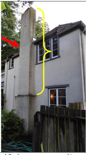
Work Item #5 - Photo 1 Replace upper masonry chimney stack to make seismic safe (yellow bracket) (visually "like for like"). Lower fire box remains. Red arrow depicts a large horizontal crack. Chimney leaning towards roof.
