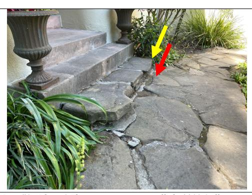
Work Item #1 - Photo 1 The stone step was installed ~2011 (yellow arrow) and pathway (red arrow) were originally level in 2002. The vertical displacement depicts significant and continued ground settling. Install support foundation under the house.
