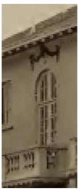
Work Program Item #2 Figures C and D: Eastern-most (left) cantilevered balconette partially obscuring large fanlight, square fixed window, and rectangular fixed window. French windows with an incorporated semicircular arch were featured in the original design (right)
