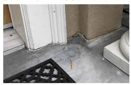
Work Program Item #1, Figures A and B: Separation of the concrete stairs from the residence foundation as a result of soil shifting to the rear slope (left). Sinking of the entry walkway and separation of the front porch as a result of general movement of earth to the west and south (right).
