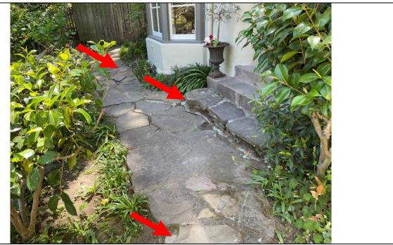
Work Item #4 - Photo 3 Red arrows show missing and or significant separation based on ground settling.
