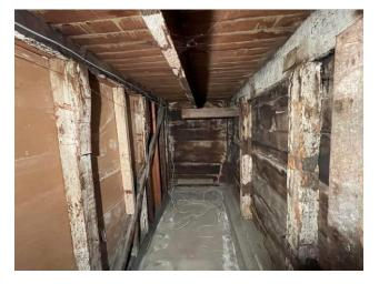
Work includes anchoring mudsills to the foundation, installing shear walls and shear transfer ties, and blocking in floor framing.
