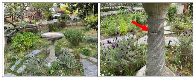
Work Item #2 - Photo 4 &5 Early if not original bird bath to be repaired. Red arrow is a crack on the pedestal post.
