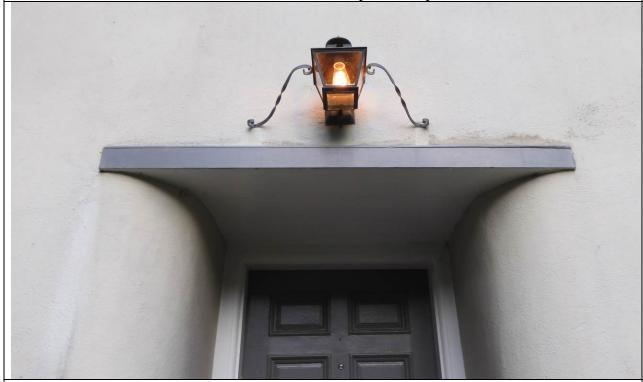
Work Item #2 - Photo 6 Remove repair and rewire original light feature. Exposed wire insulation present. Patch and paint exterior wood and stucco.
