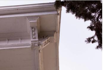
Observe rotted and deteriorated bracket. This damage is typically painted over throughout the house.
