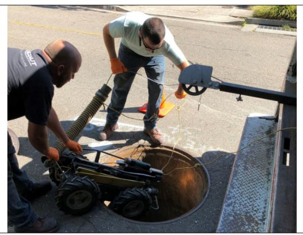
Work Item #1 - Photo 2 Robot with camera entry into Trestle Glen Road culvert access port directly in front of 901 Trestle Glen Road (2019).
