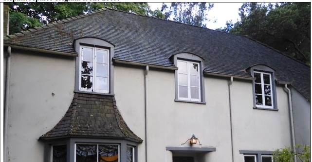
Work Item #4 - Photo 1 Replace wood shingle rood with new fire-retardant rated wood shingle roof on upper & lower portions. Wood roof dated early 1990s.
