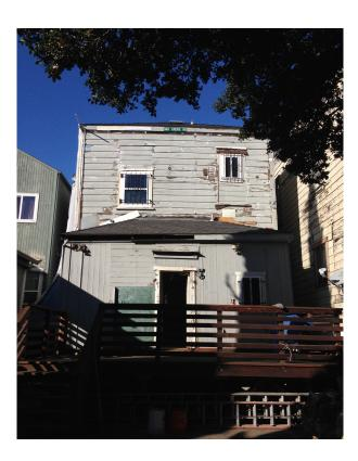
The siding is warped, and the paint is deeply blighted on the south and east sides. The rear of the house is dilapidated and rotten.
