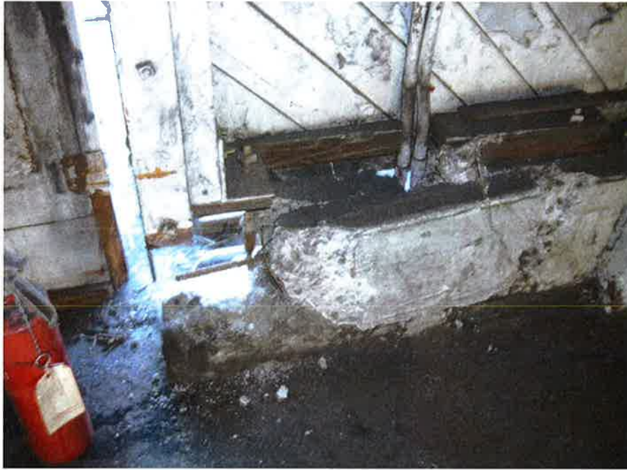
Photo 7: Damaged Stem Wall at Door
