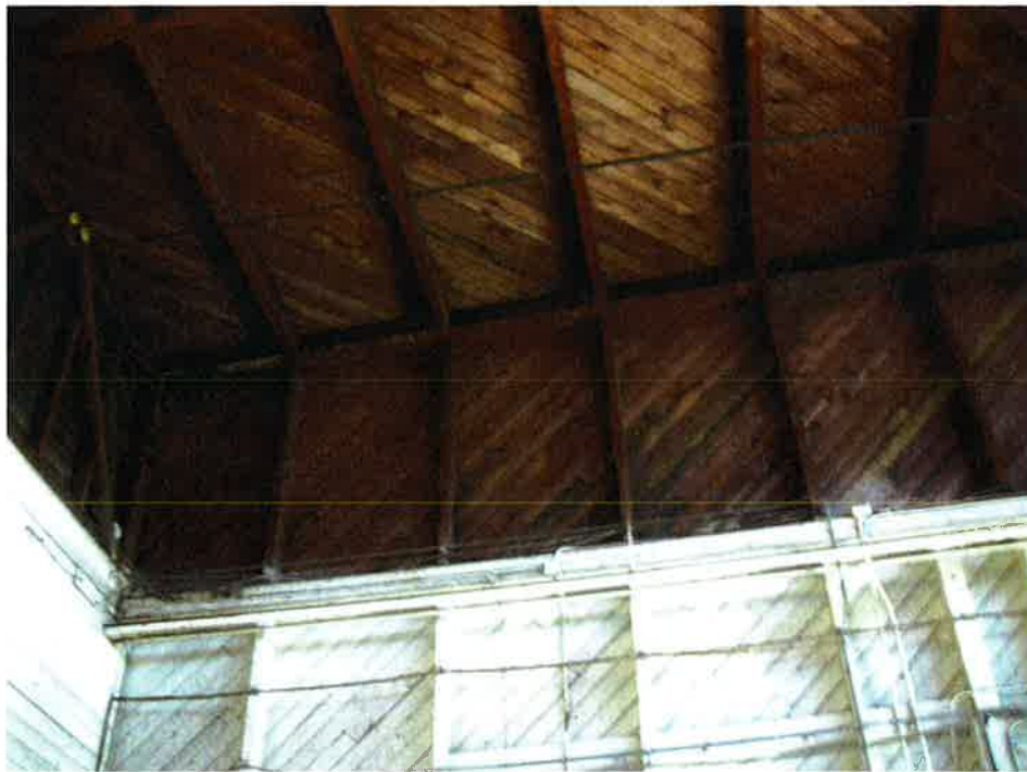
Photo 5: Wall/Roof Sheathing
