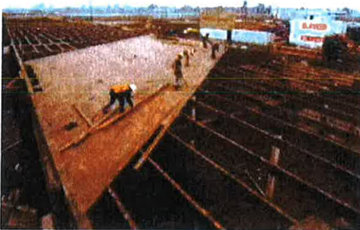
Figure 5.1- Roof sheathing removal
