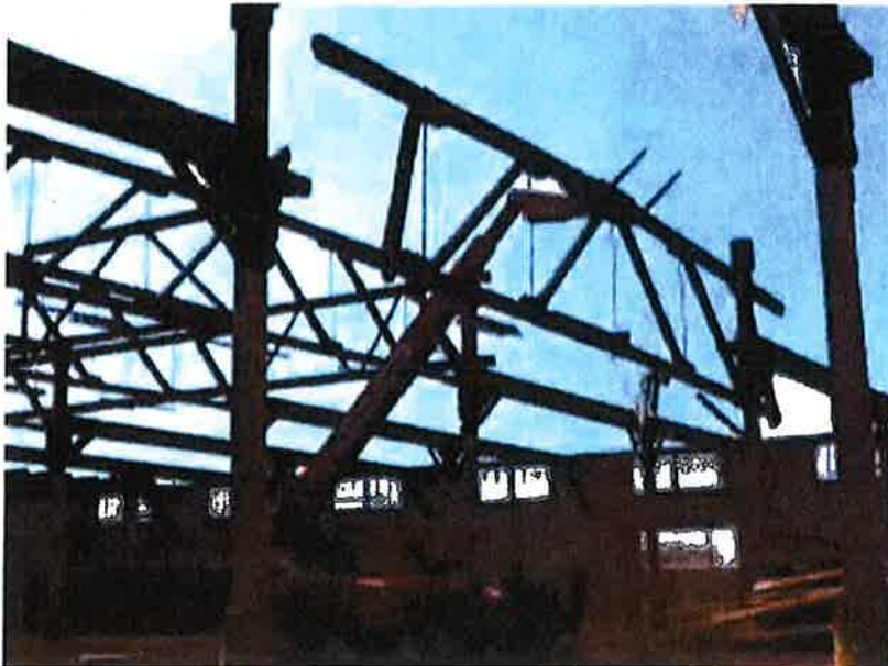
Figure 5.7 Truss removal
