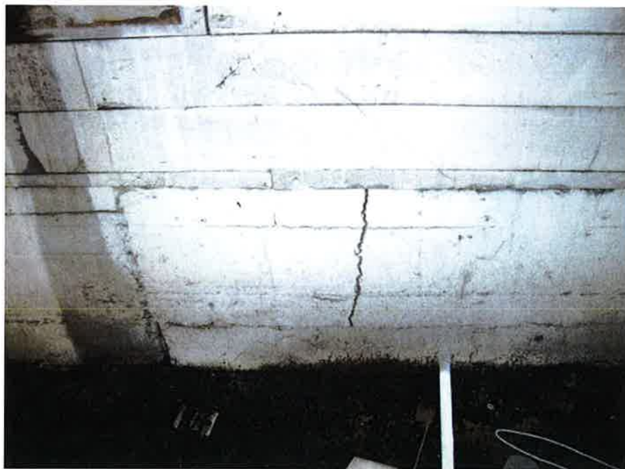
Photo 9: Cracking at Stem Wall (Interior)
