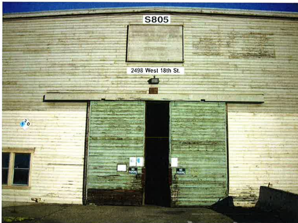
Photo 13: Weathered Siding
