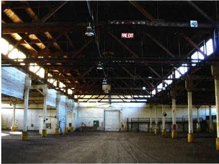
Photo 3: Roof Truss at Clearstory
