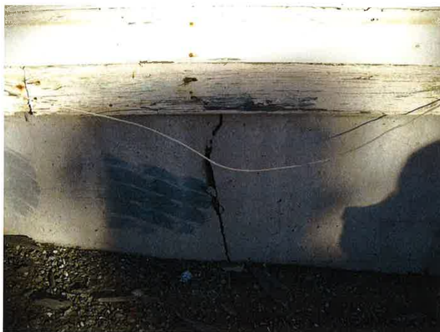
Photo 10: Cracking at Stem Wall (Exterior)
