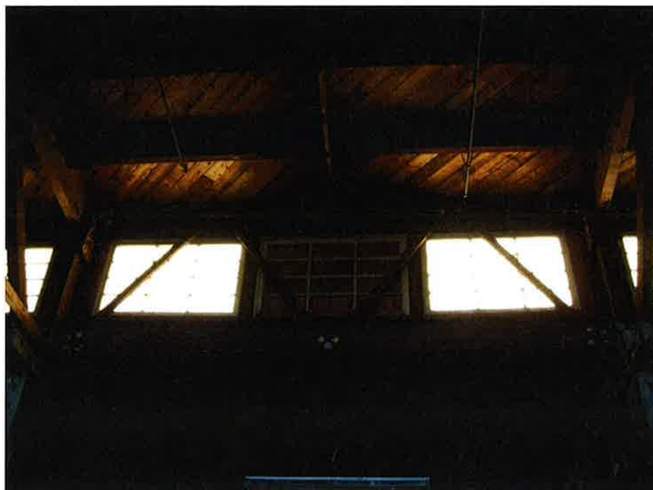
Photo 6: Clearstory Bracing
