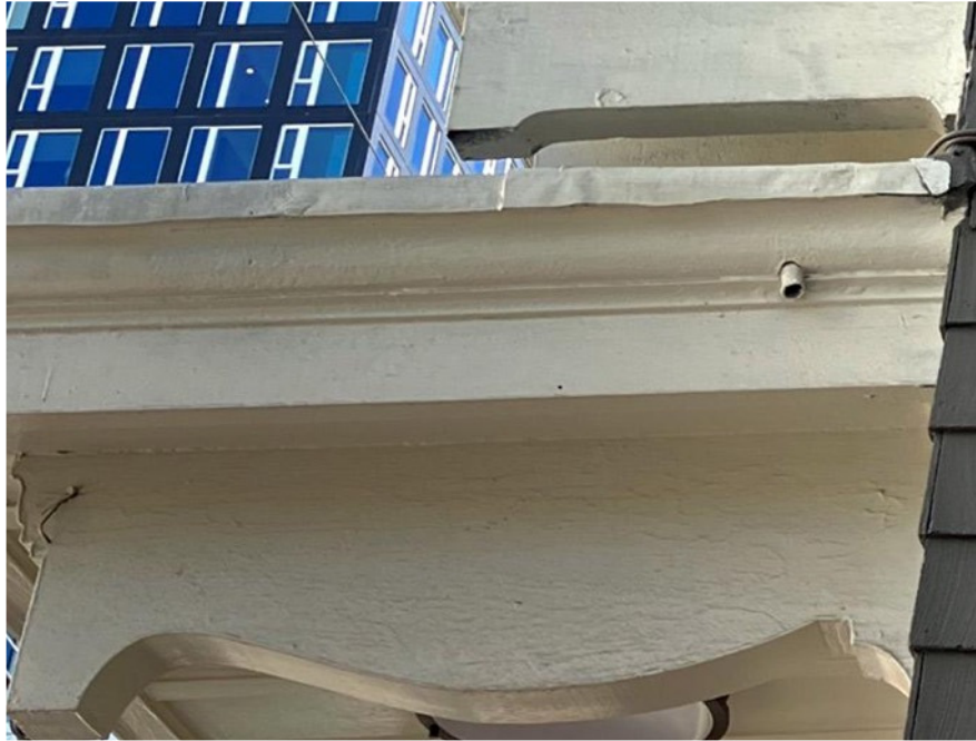
Photo #7 - Overhang with sheet metal covering
