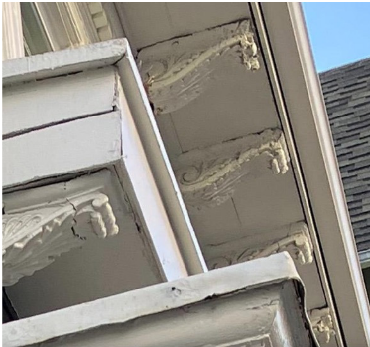
Photo #8 – Flower Box and Eaves Corbels
