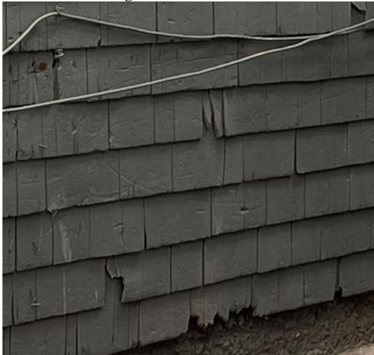
Photo #11 - Shingles on west side of house
