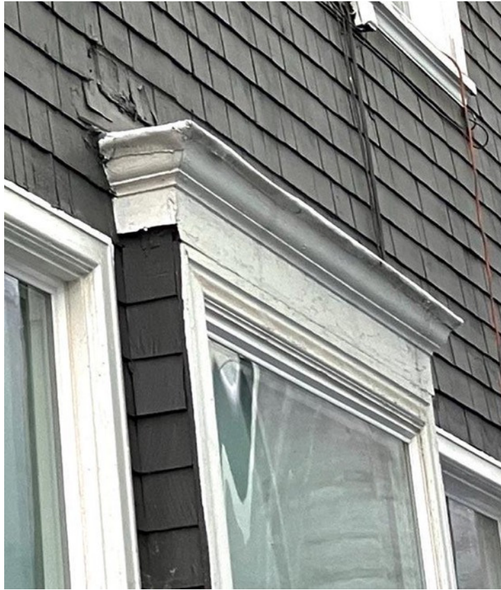
Photo #4 - Window Cornice
