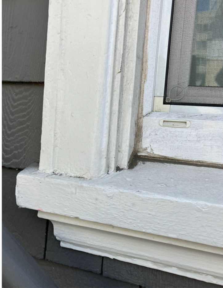
Photo #2B: Close-up of original trim from lower façade window
