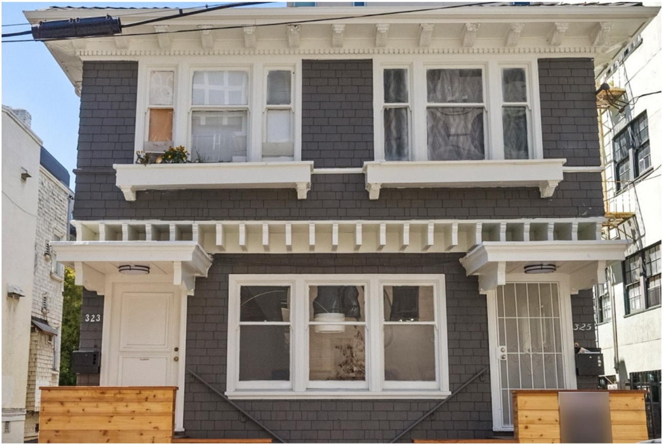
325 24th Street Facade with all Original Windows
