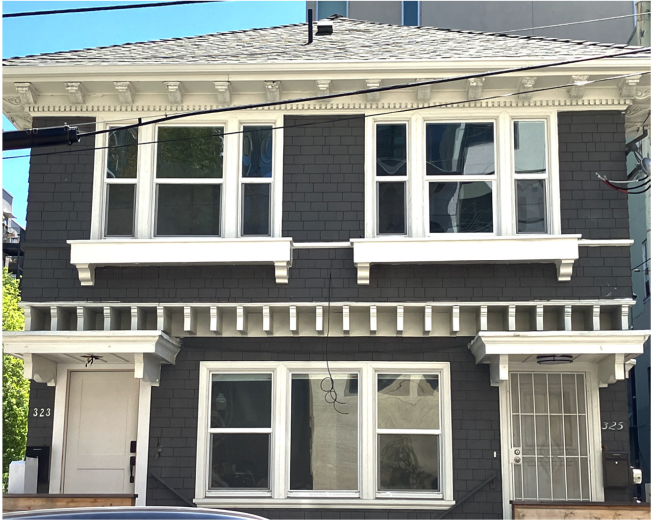
325 24th Street Current Facade with new Vinyl Windows and new flower box corbels
