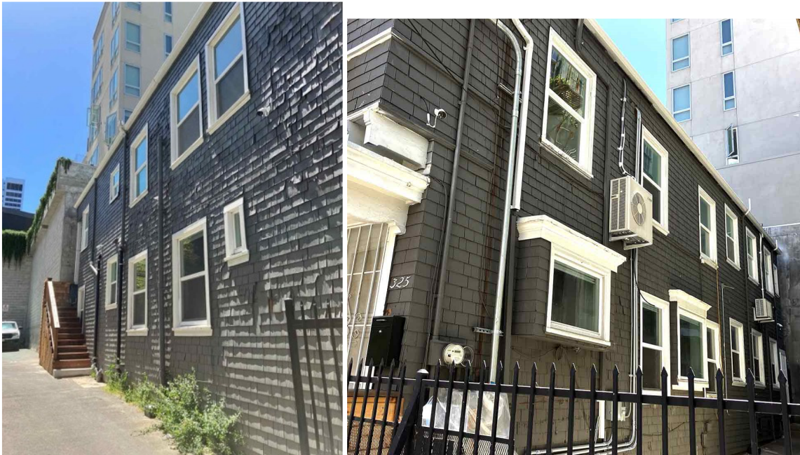
East side (left) and west side (right) of house
