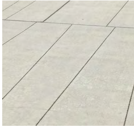
1. CIP Concrete Paving - Finish 1 Pedestrian and Vehicular
