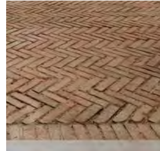
4. Site Salvaged Brick Paving
