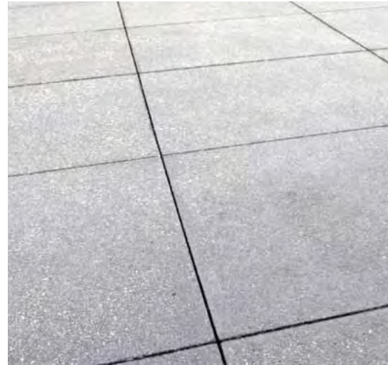
3. CIP Concrete Paving - Finish 3 Pedestrian
