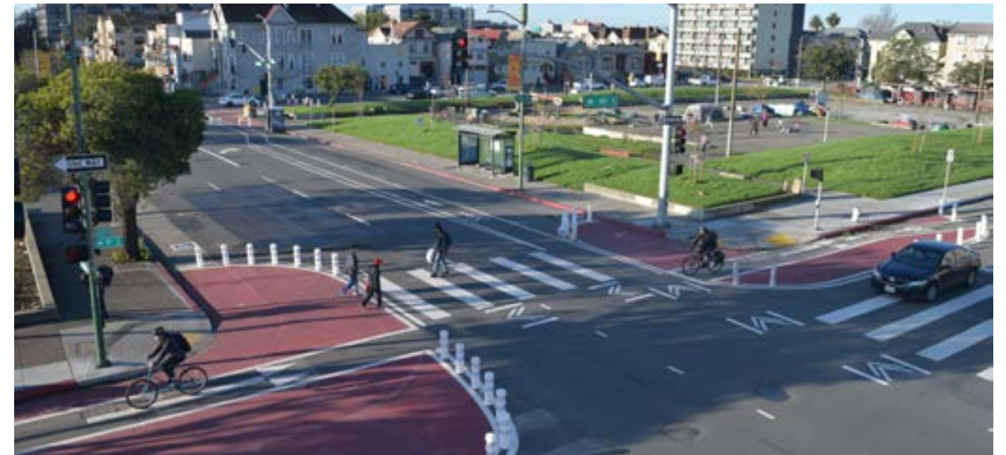
Intersection crossing improvements at 9th Street and Madison Street (Lake Merritt BART)
