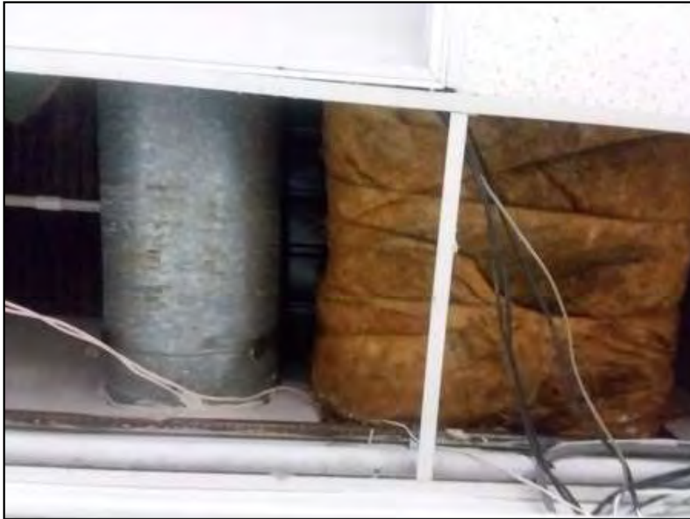
7 : 2716 International Boulevard - Exposed HVAC air duct.
