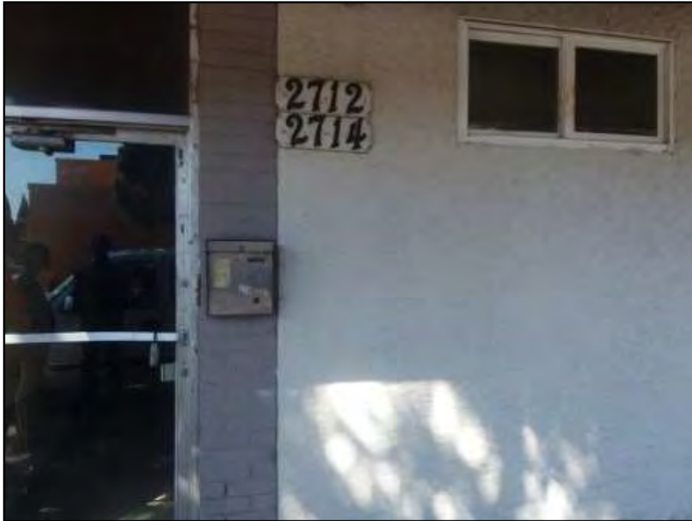
13 : Exterior of 2712-2714 International Boulevard.
