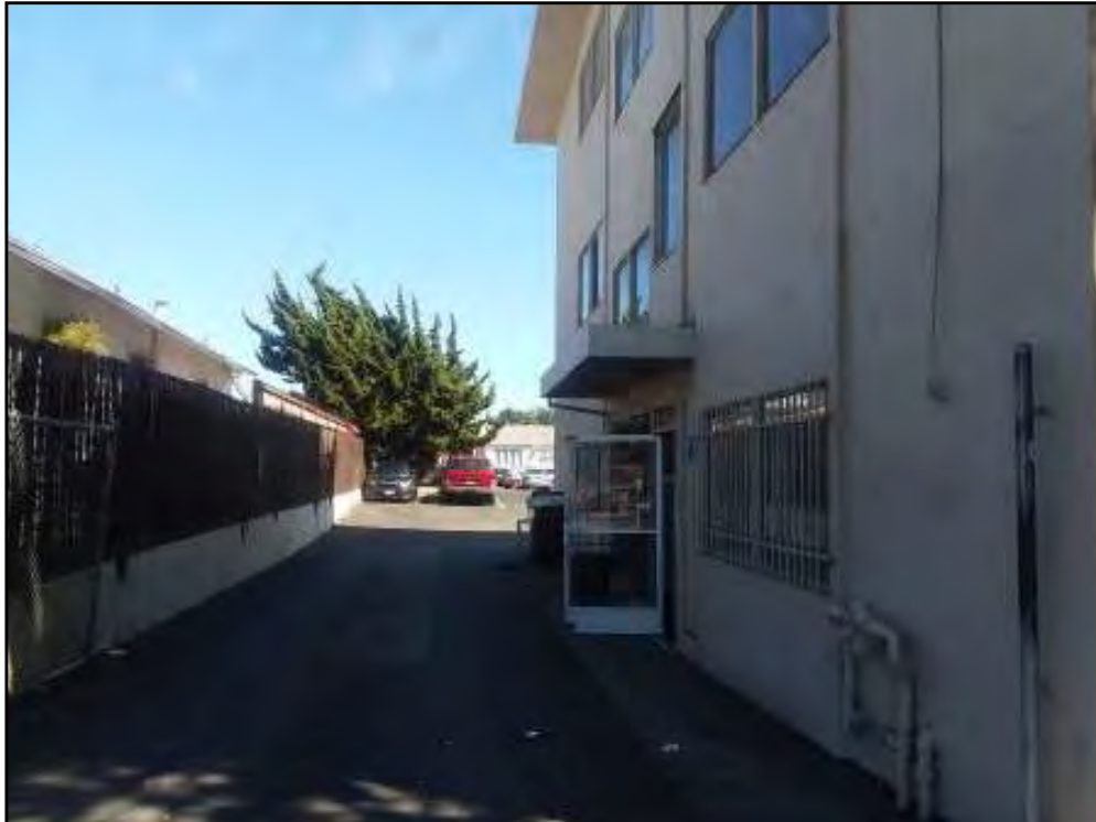
18 : 2700 International Boulevard - Exterior photo of building oriented towards the southeast.
