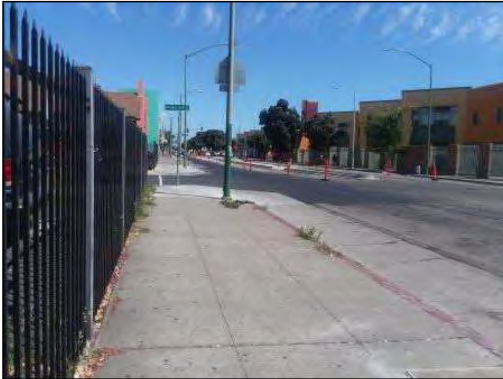
15 : 1409,1415 International Boulevard - Oriented towards the southeast along International Blvd.
