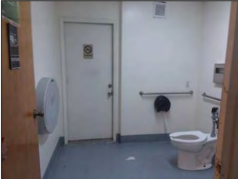
4 : 2700 International Boulevard - First floor bathroom
