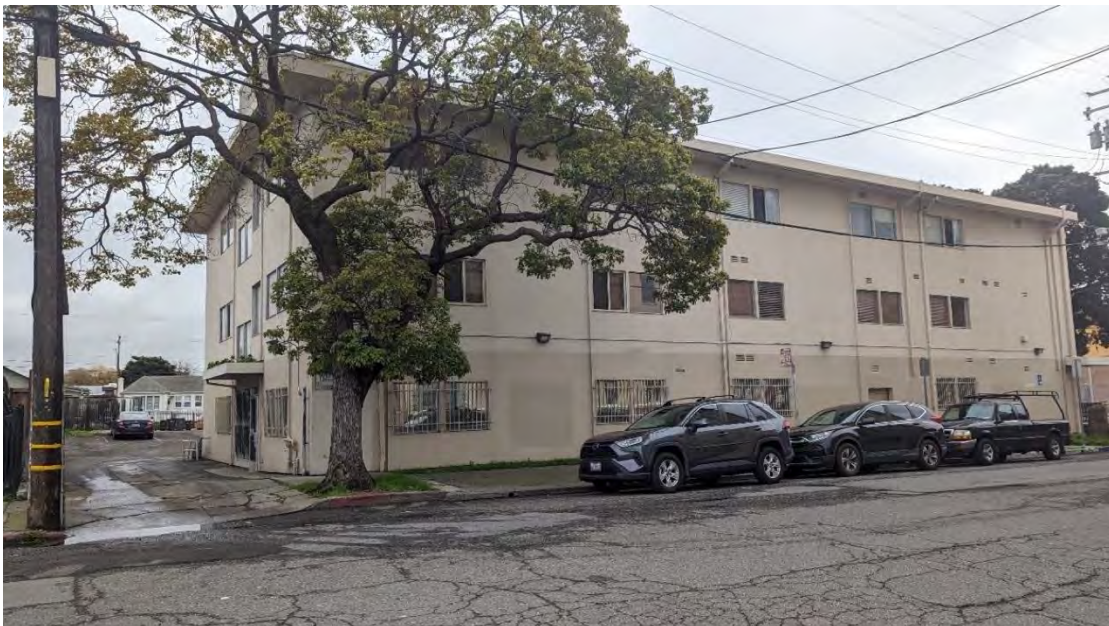
Figure 46. North and west elevations, facing southeast.
