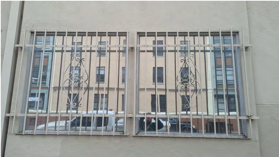
Figure 45. Paired windows with metal window grille.
