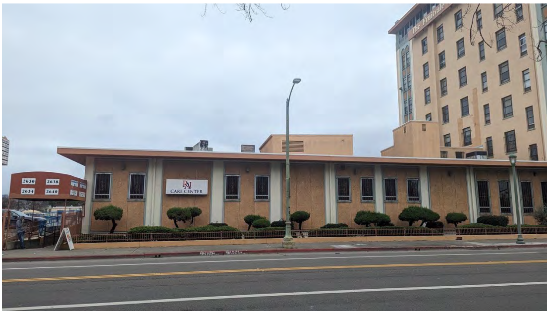
Figure 2. South elevation of ca. 1988 addition.
