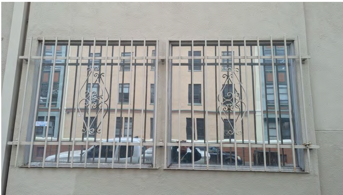
Figure 4. Paired windows with metal window grille.
