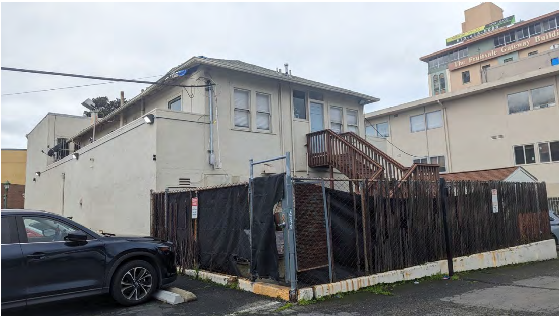
Figure 5. North and east elevations, facing southwest.
