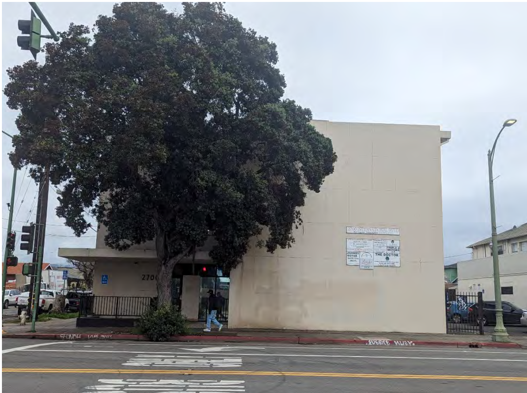
Figure 1. South elevation, facing north.
