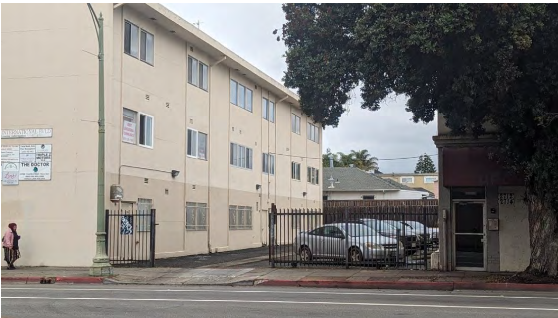
Figure 10. East elevation, showing the building (left) and parking lot, facing northwest.
