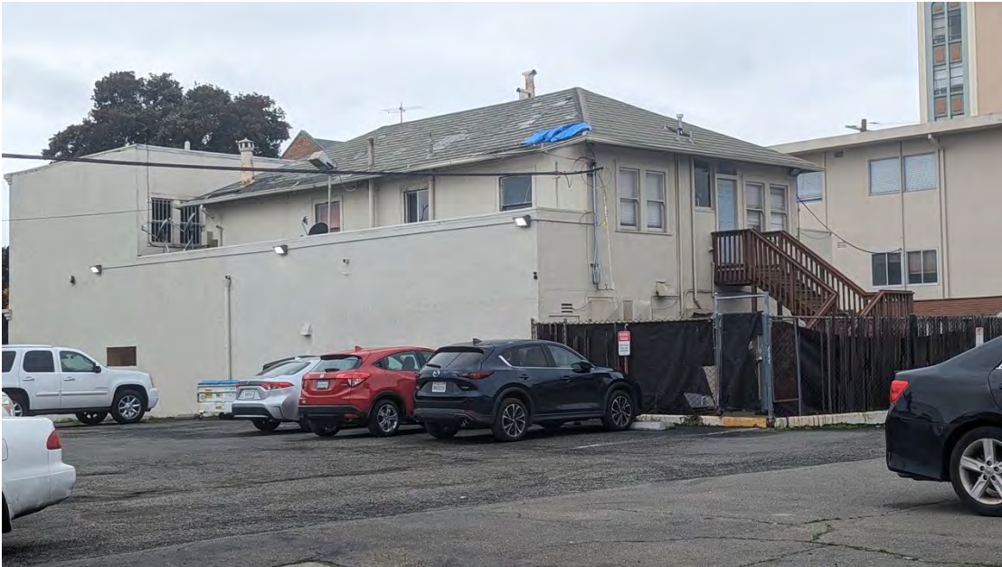
Figure 6. North and east elevations, facing southwest.
