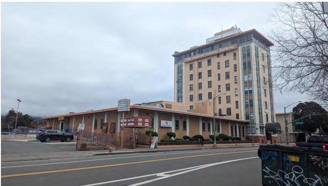
Figure 66. South and west elevations, facing northeast.
