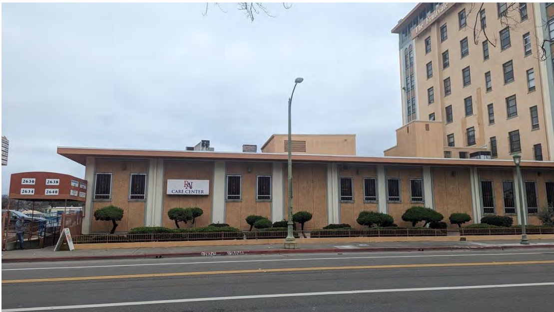
Figure 65. South elevation of ca. 1988 addition.
