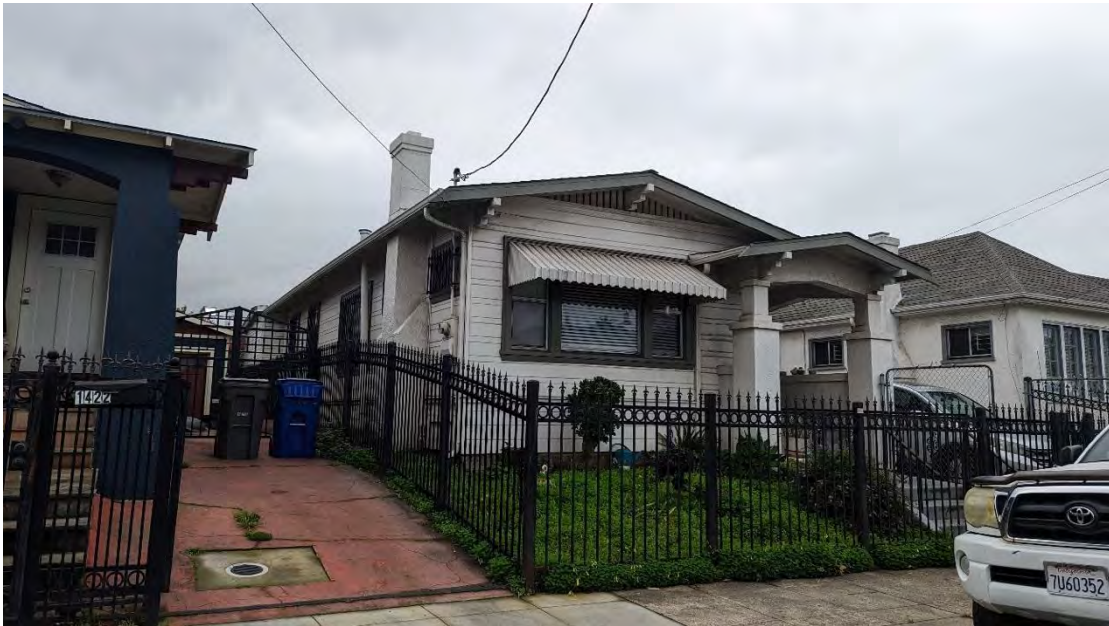
Figure 75. North and west elevations, facing southwest.
