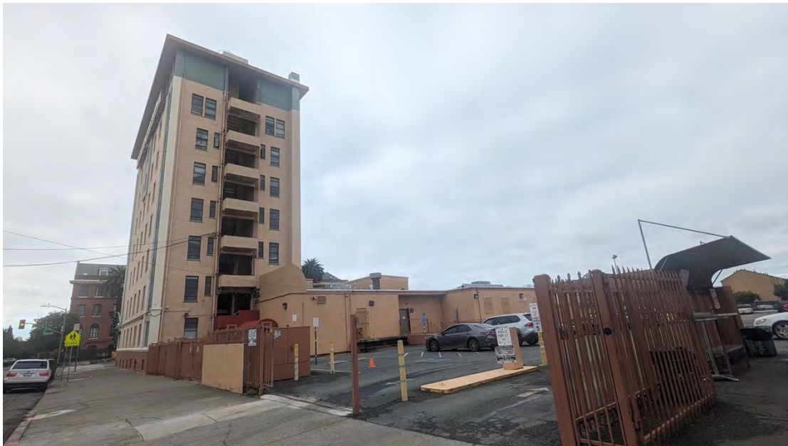
Figure 5. East and north elevations, facing southeast.
