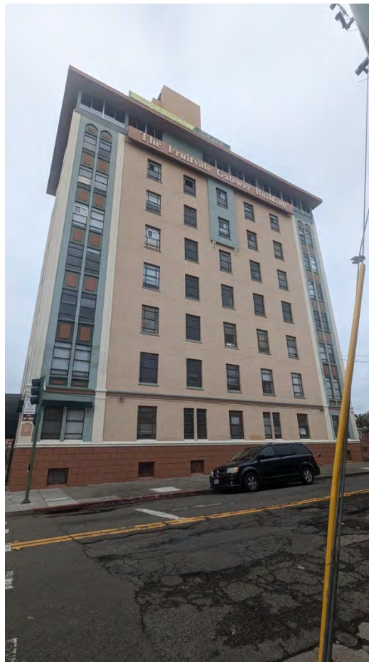
Figure 7. East elevation, facing west.
