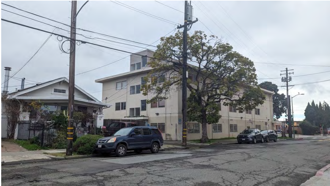
Figure 6. North and west elevations, facing southeast.
