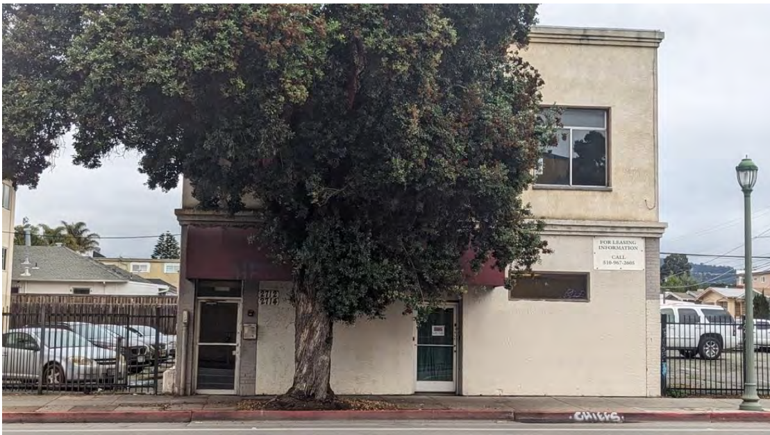
Figure 52. South elevation, facing north.
