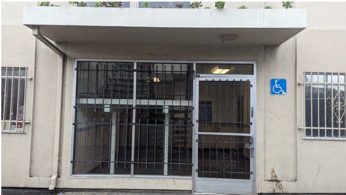
Figure 7. The entrance is on the north elevation, facing south.
