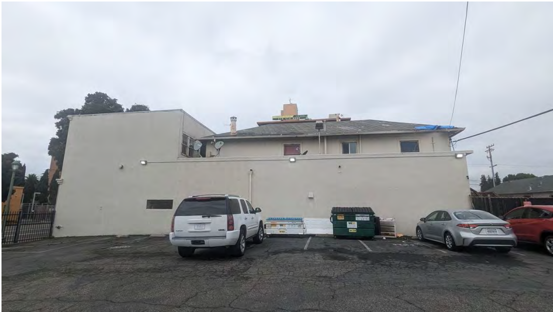
Figure 59. East elevation, facing west.
