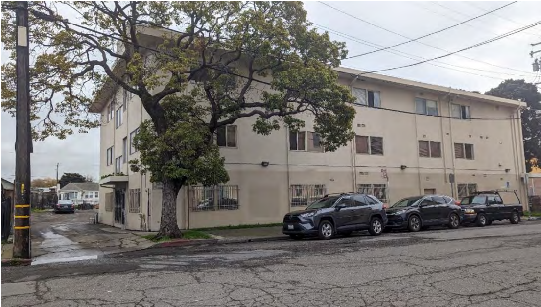
Figure 5. North and west elevations, facing southeast.
