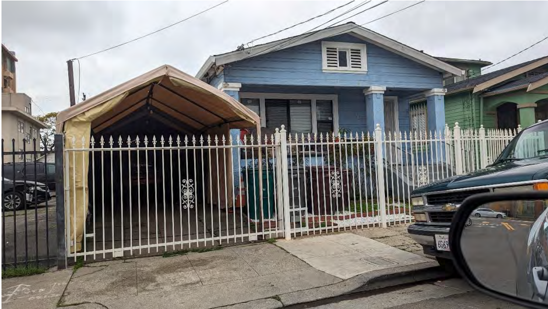
Figure 73. East elevation, facing west.
