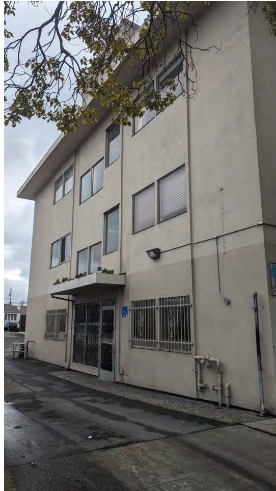
Figure 49. North elevation, facing southeast.
