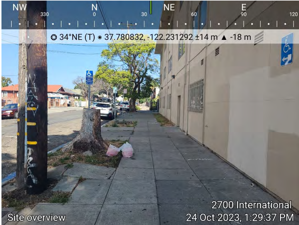
Figure 36: Overview of western exterior boundary of the Project Area where soil is exposed.
