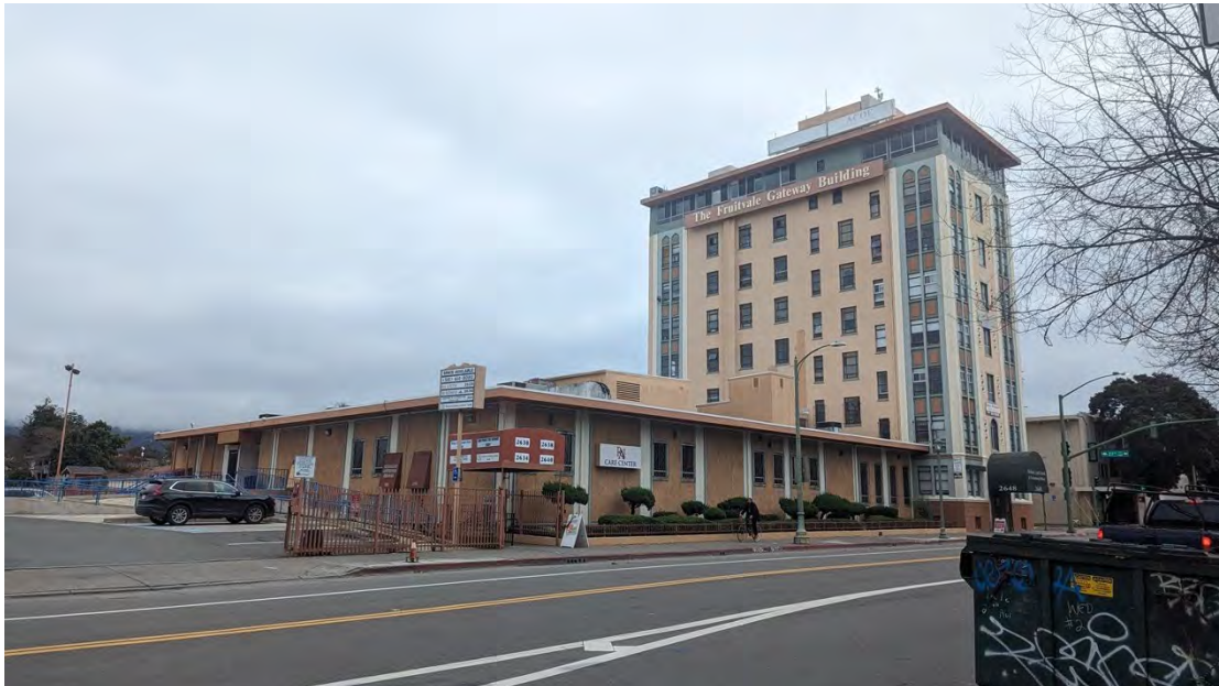
Figure 3. South and west elevations, facing northeast.
