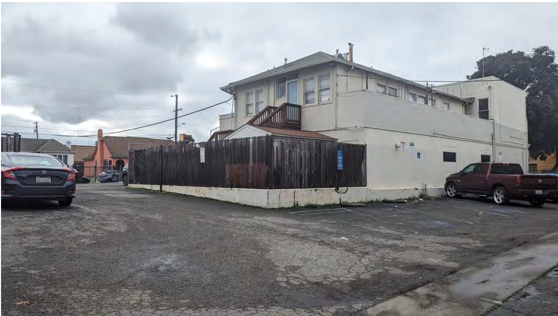
Figure 3. North and west elevation, facing southeast.
