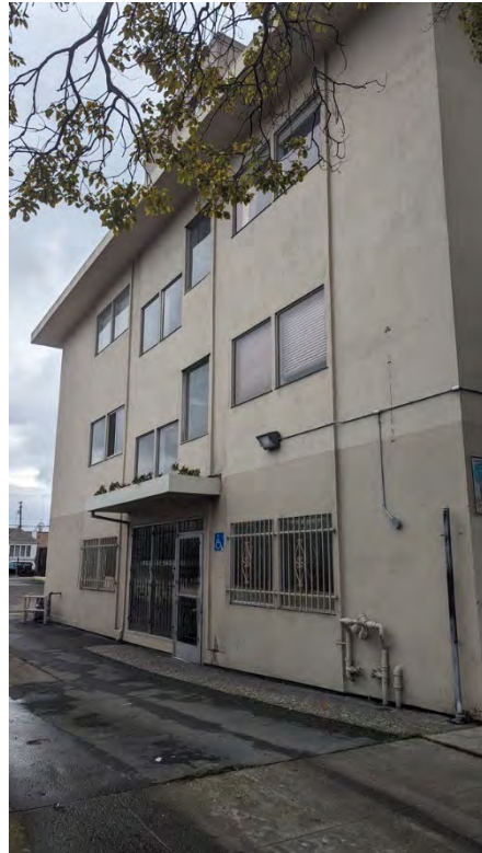
Figure 8. North elevation, facing southeast.
