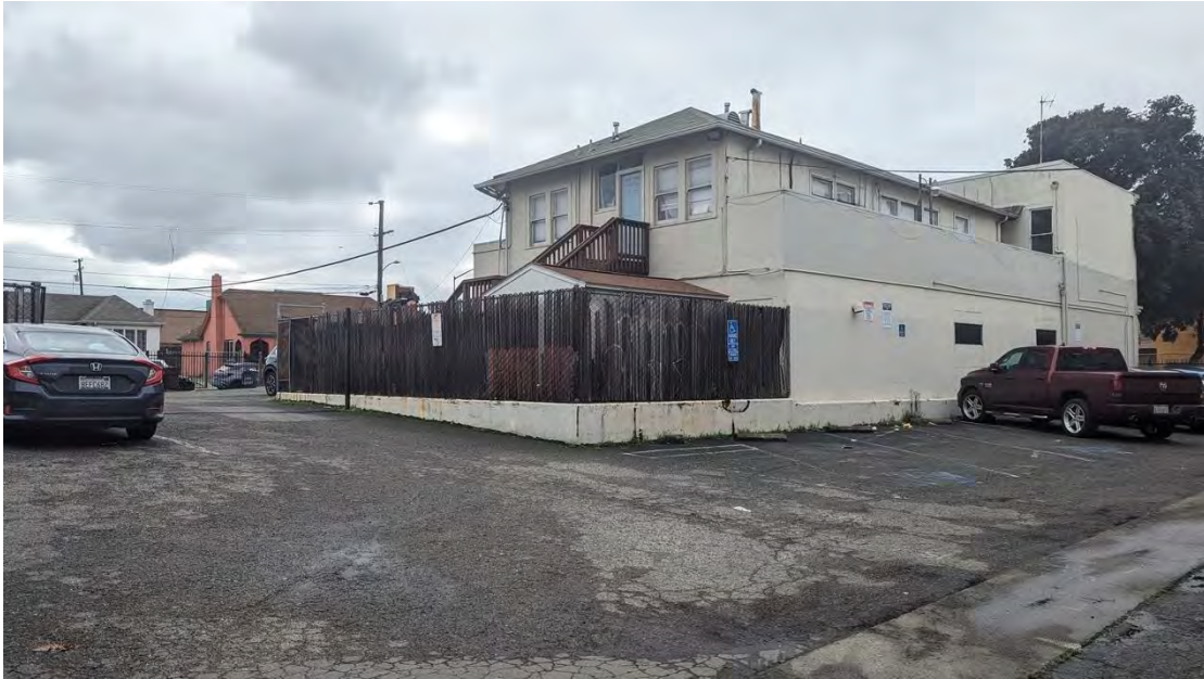
Figure 55. North and west elevation, facing southeast.
