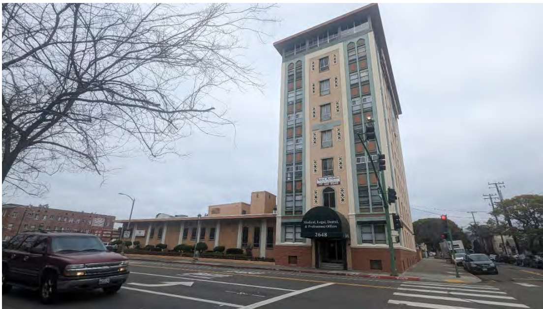
Figure 1. South elevation, facing north.
