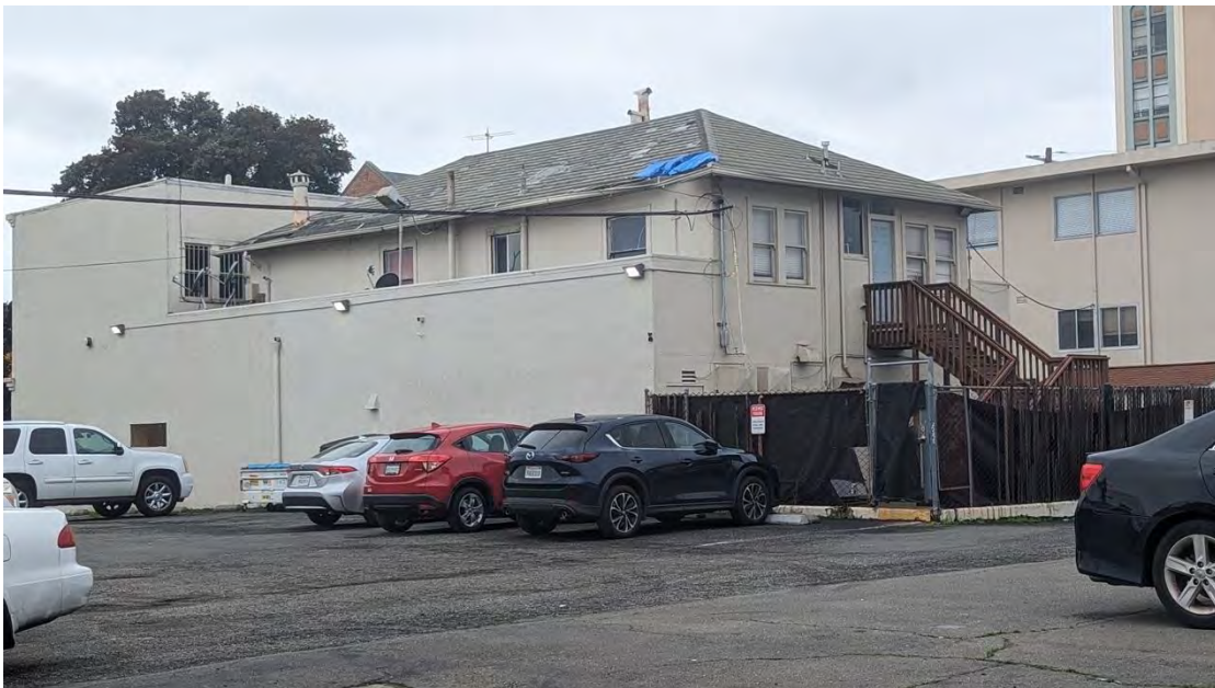
Figure 58. North and east elevations, facing southwest.
