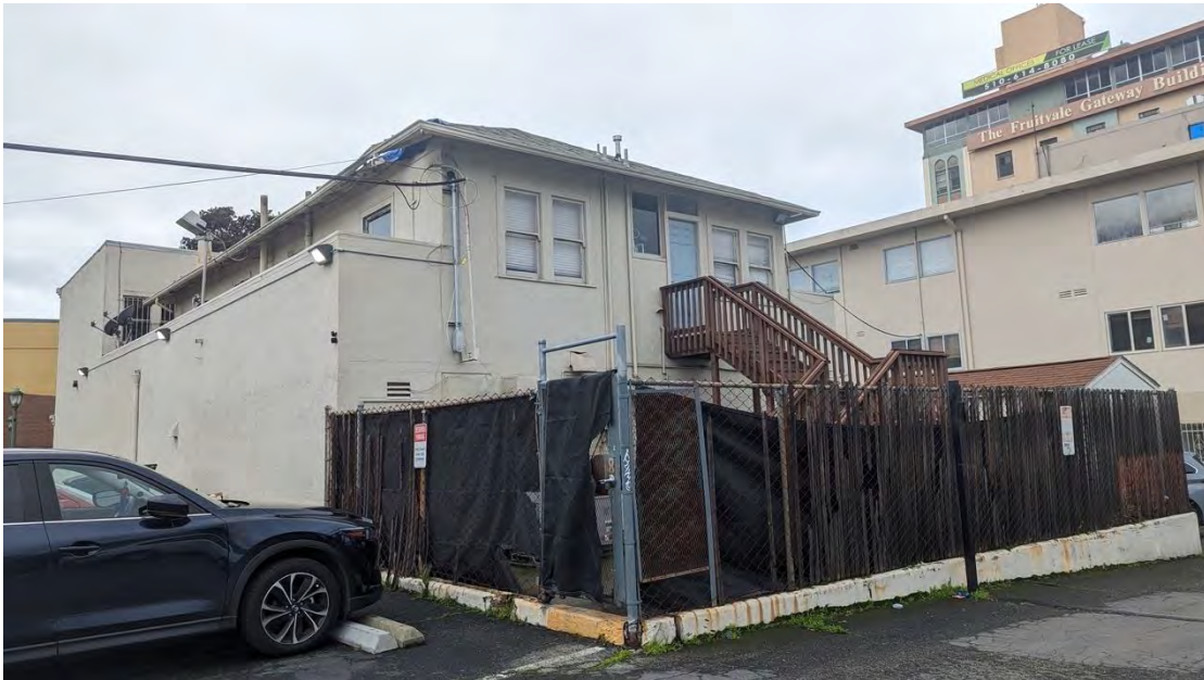
Figure 57. North and east elevations, facing southwest.
