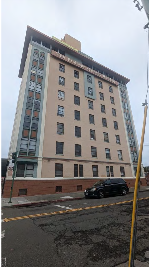
Figure 70. East elevation, facing west.
