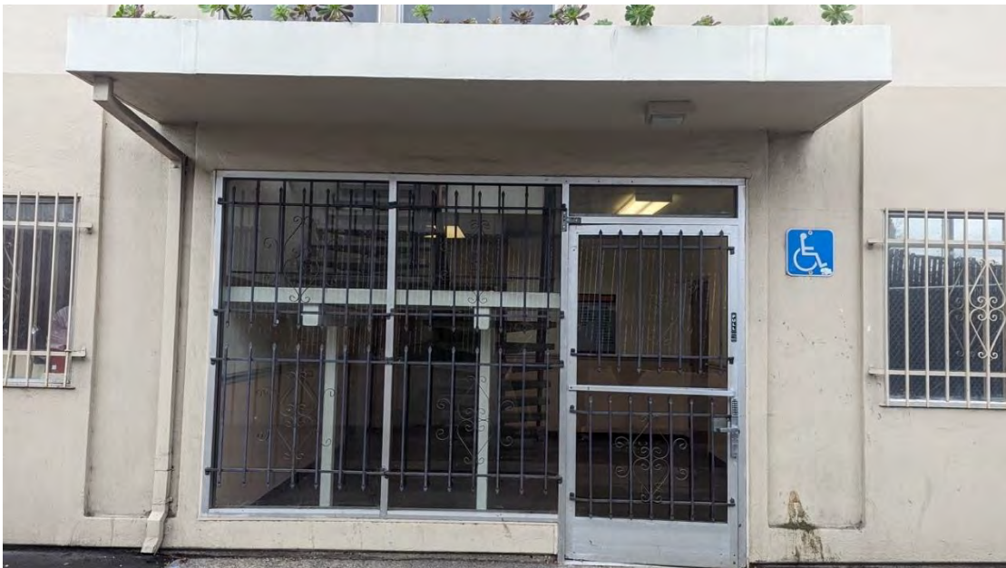
Figure 48. The entrance is on the north elevation, facing south.
