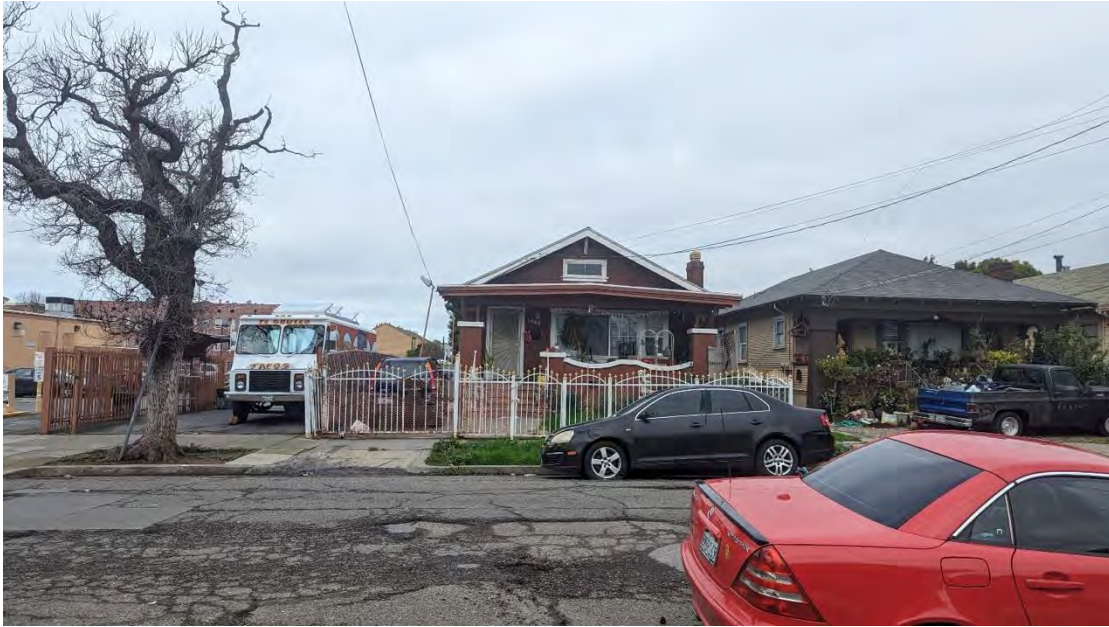
Figure 71. East elevation, facing west.
