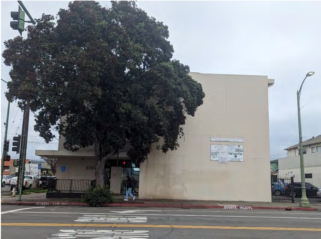
Figure 42. South elevation, facing north.
