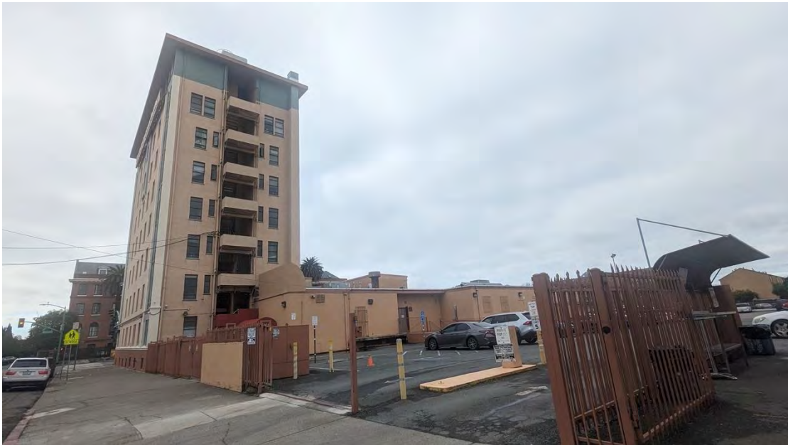
Figure 68. East and north elevations, facing southeast.
