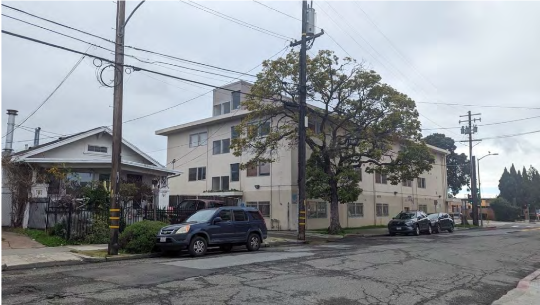
Figure 47. North and west elevations, facing southeast.
