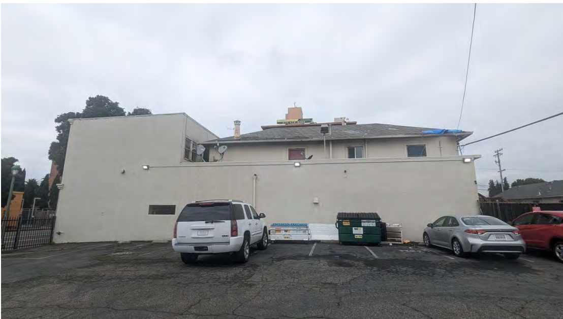
Figure 7. East elevation, facing west.
