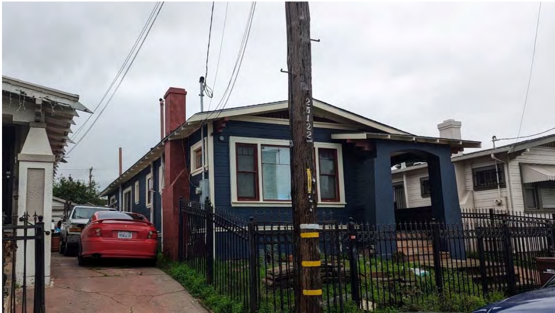
Figure 74. North and west elevations, facing southeast.
