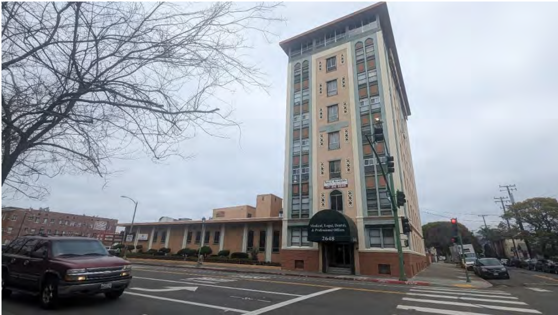
Figure 64. South elevation, facing north.
