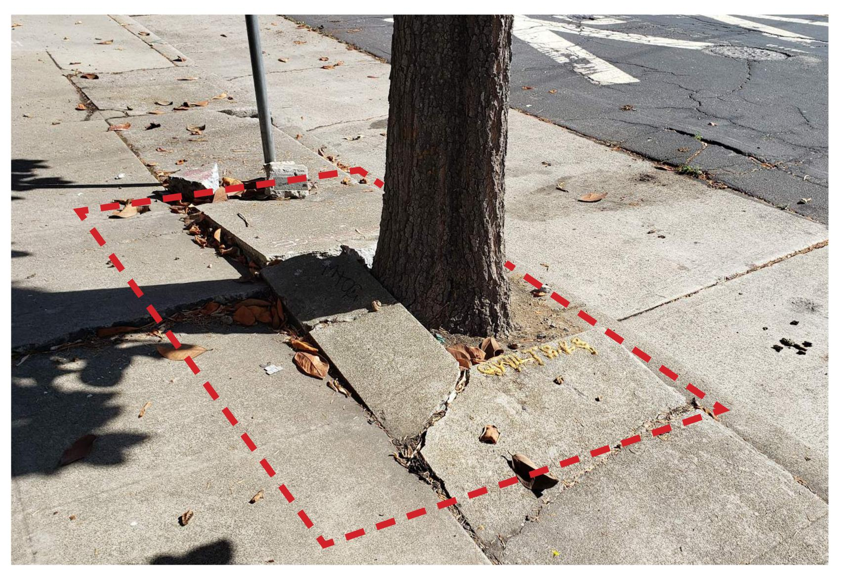
TREE TO BE PRESERVED. SIDEWALK DAMAGE CAN BE CORRECTED BY ENLARGING TREE WELL TO LINE SHOWN IN RED.
