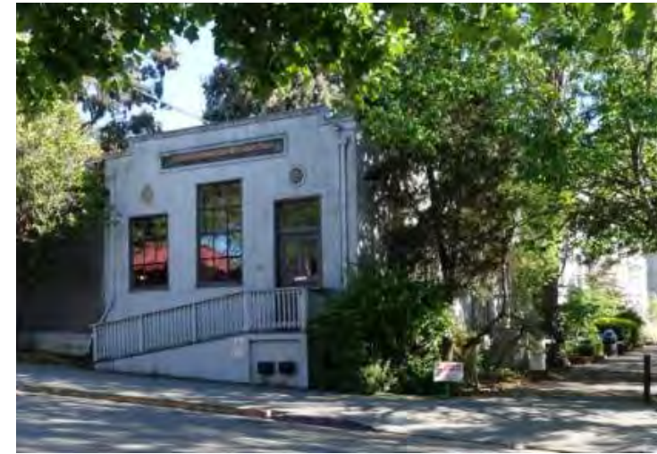
06 | Facilities Building on Clifton
