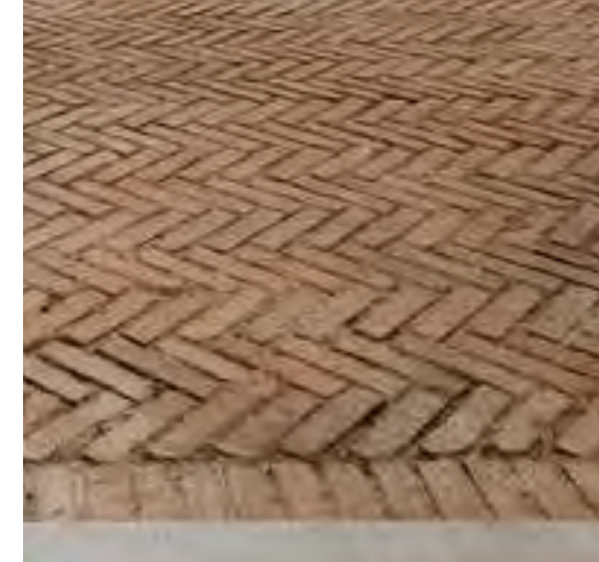
4. Site Salvaged Brick Paving
