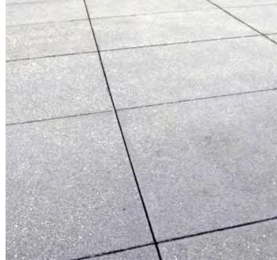
3. CIP Concrete Paving - Finish 3 Pedestrian
