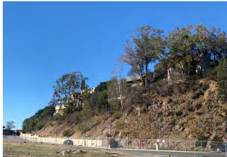
03 | View of Site and Access Road from Southeast
