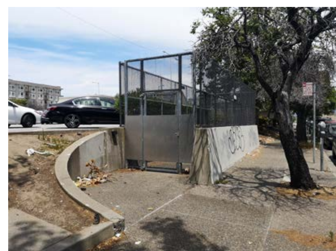
STAIR: TO REMAIN FINAL DESIGN TREATMENT TO BE DEVELOPED WITH BART. OPPORTUNITY FOR ART.
