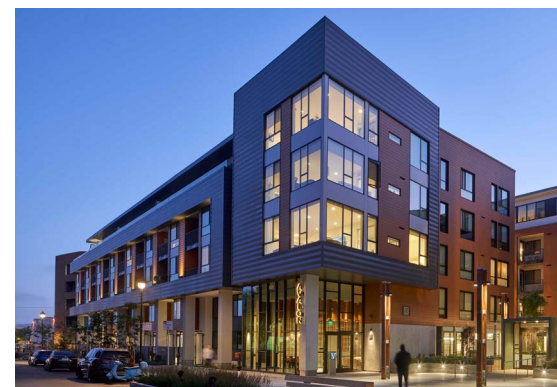
Figure 24: Building Corner at 8th and Fallon Streets
