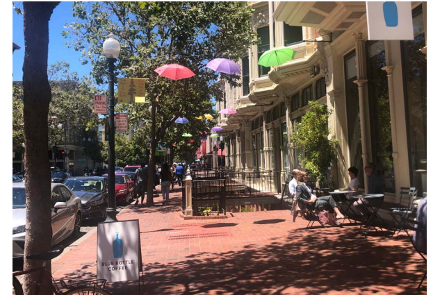
Figure 27: Festival Lighting Infrastructure Cables
