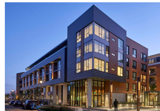
Figure 24: Building Corner at 8th and Fallon Streets
