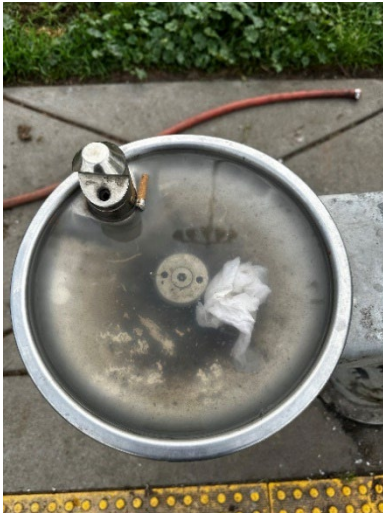
Nonfunctioning and clogged water fountain
