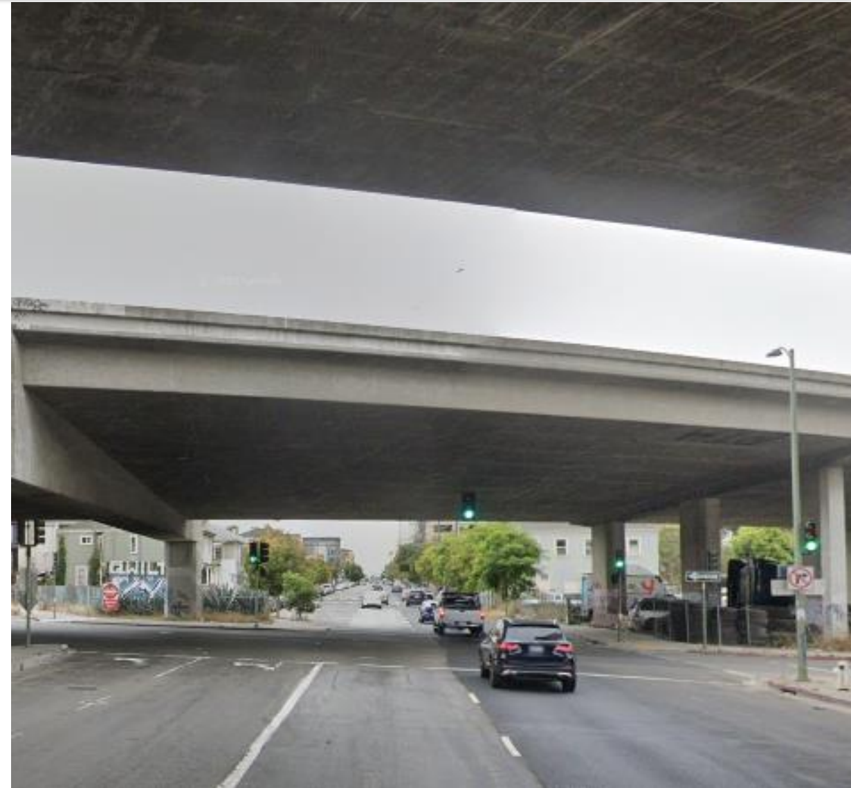
7 th St, under I-980, Brush St, looking east
