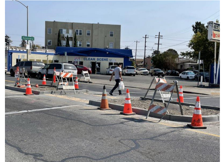
Pedestrian Island Construction on Bancroft and Avenal (2021)
