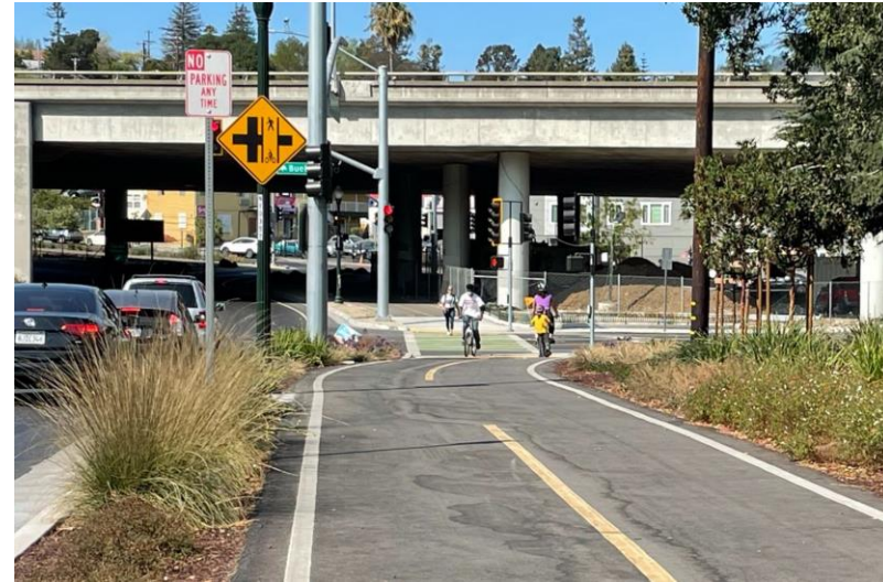
LAAMPS Project at MacArthur Blvd & Richards Road (completed 2021)
