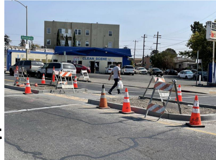
Pedestrian Island Construction on Bancroft and Avenal (2021)
