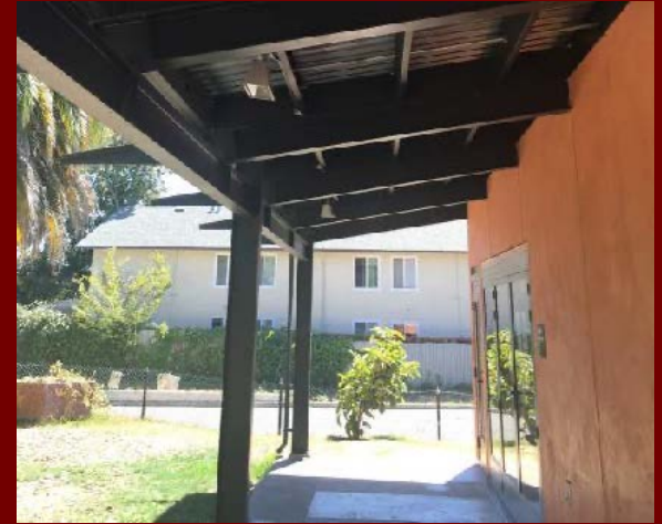
Covered Walkway around the Center for History and Community
