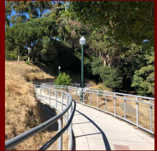
ADA Ramp to Peralta Creek Nature Area
