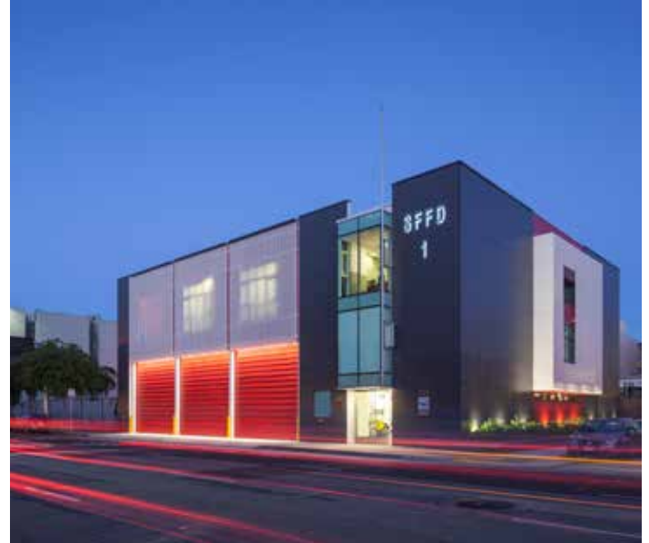
FIREHOUSE NO. 1 IN SAN FRANCISCO, CA IS A RESILIENT EMERGENCY SERVICES FACILITY.
