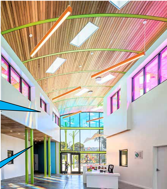
THE RAINBOW RECREATION CENTER IN OAKLAND, CA HAS AN IN-SLAB RADIANT SYSTEM.
