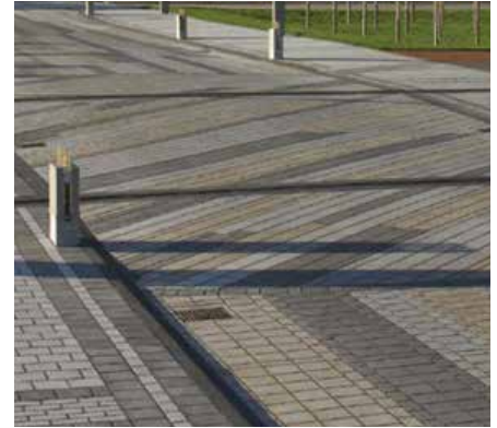
PAVERS AS FIRE ACCESS ROAD
