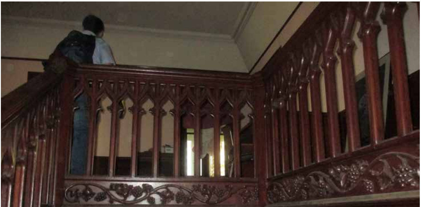
INTERIOR STAIR RAILING AT SECOND FLOOR.
