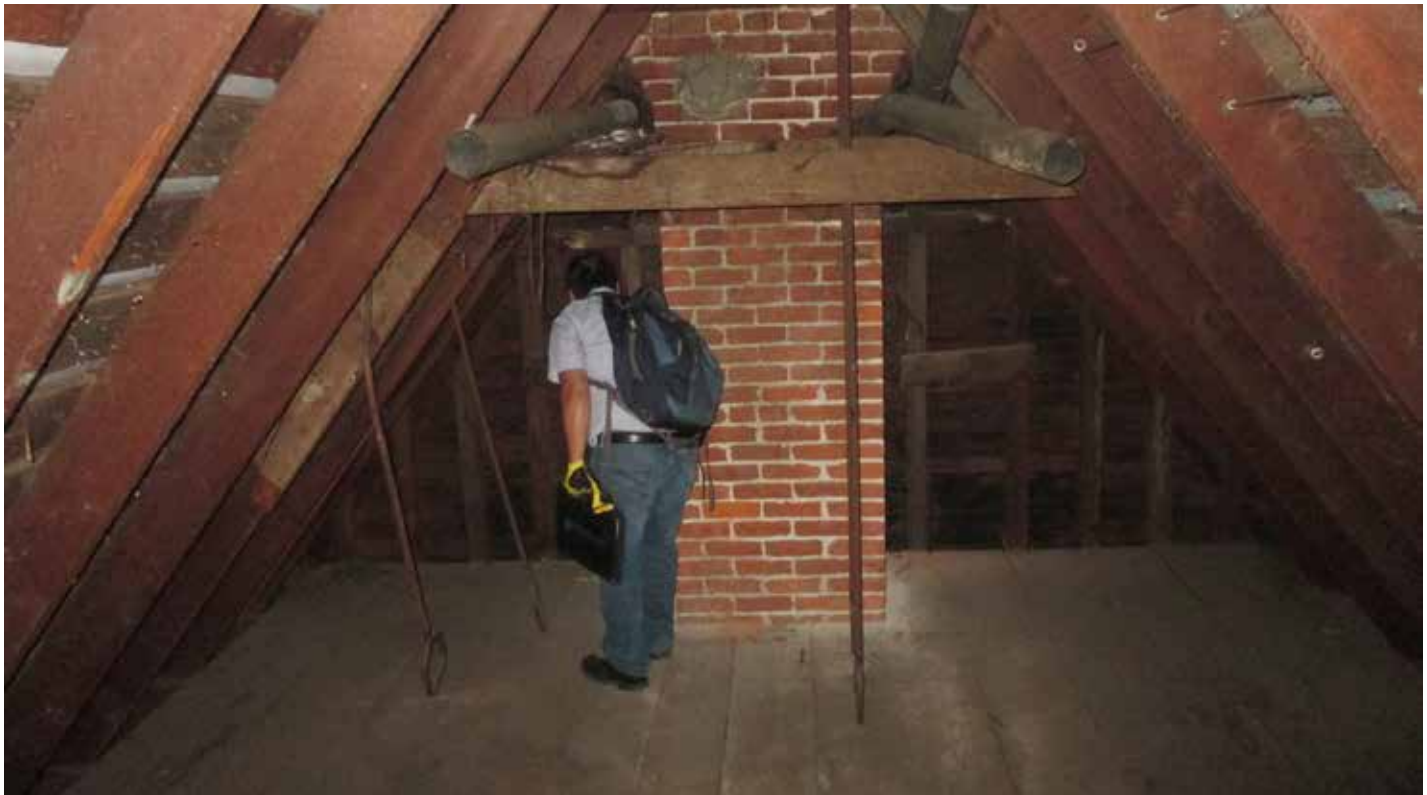
ATTIC INTERIOR WITH ARCHED BRICK CHIMNEY.
