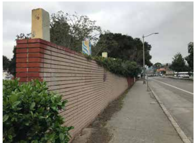
VIEW FROM BROADWAY SIDEWALK
