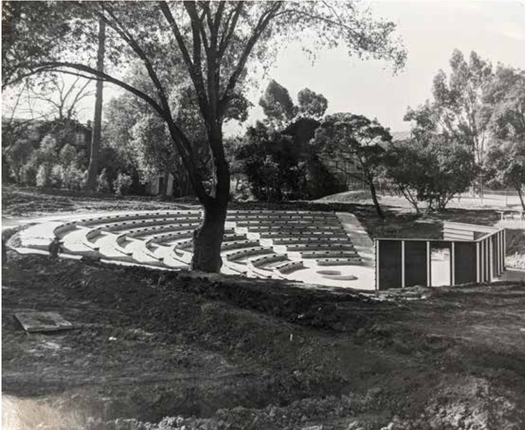
AMPHITHEATER AT COMPLETION OF CONSTRUCTION
