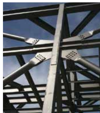
7 RESILIENT LATERAL RESISTING FRAME
