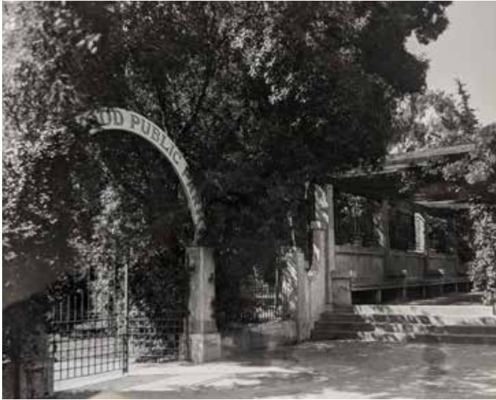
A FORMER ENTRANCE GATE ON BROADWAY
