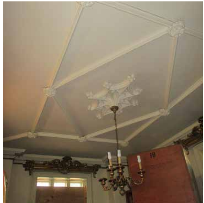
INTERIOR PLASTER CEILING MOLDING DETAIL.
