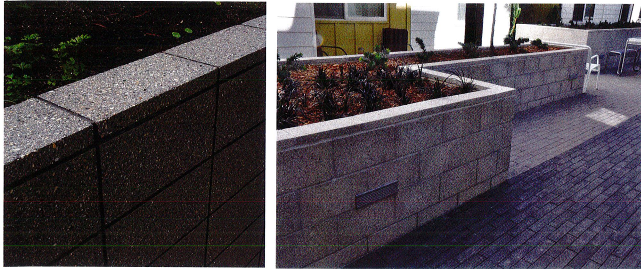
CMU BLOCK WALLS: 6" WIDE WITH GROUND FACE FINISH, DOUBLE WIDE AT SEAT WALL AREAS 16" WIDE
