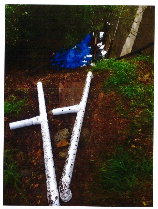
ENERGY DISSIPATERS ARE CONNECTED TO 4" FLEX STORM DRAIN LINES. THEY ARE USED TO REDUCE THE FLOW OF THE STORM DRAIN WATER. A FLEX LINE IS CONNECTED TO THE END OF THE DISSIPATER AND WATER TRICKLES THROUGH THE HOLES IN THE PIPE DISPERSING THE WATER. THESE DISSIPATERS WILL BE LOCATED OVER THE RIP RAP INSTALLED. THESE ARE THE DISSIPATERS THAT WERE WASHED AWAY AND RECOVERED.
