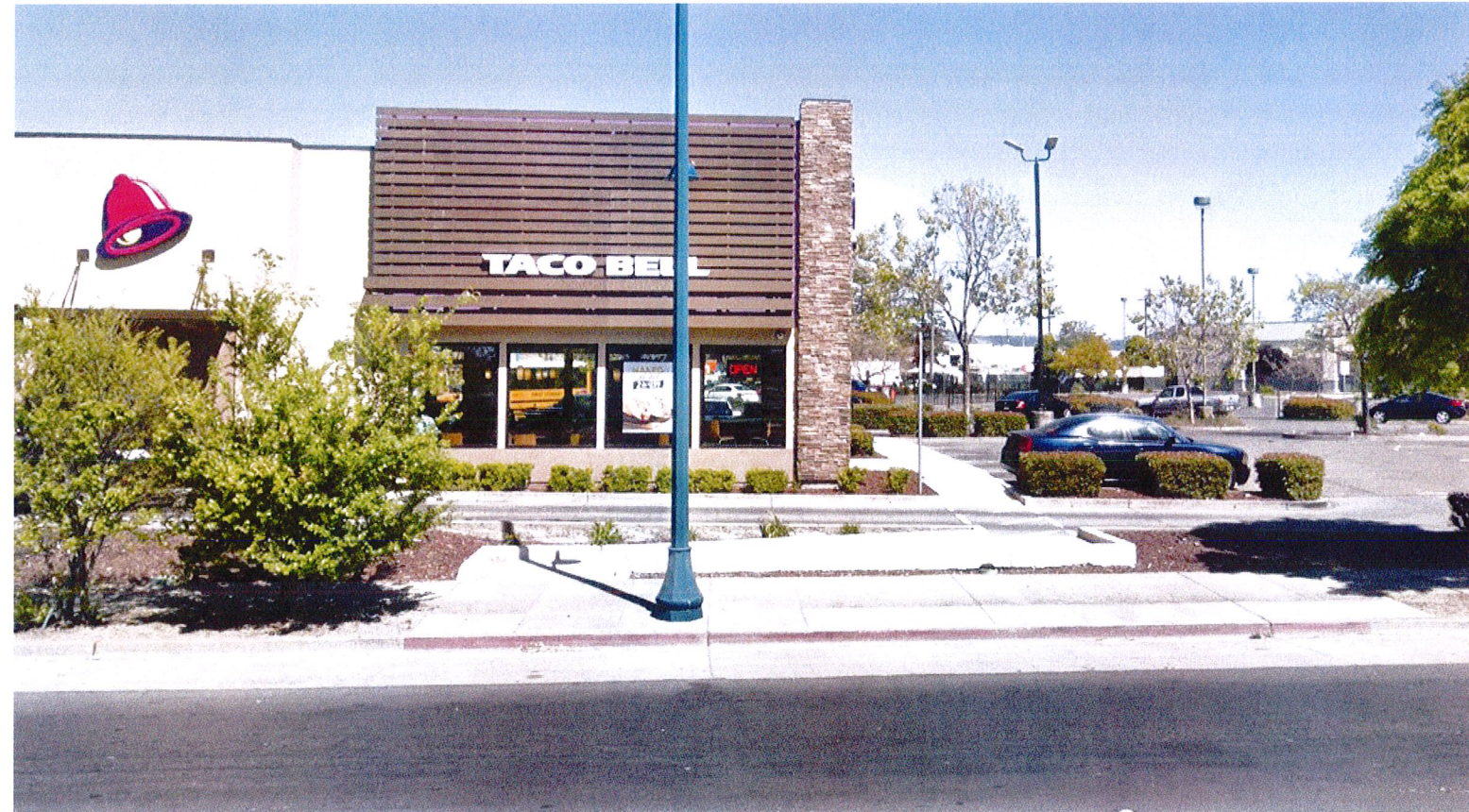
EXISTING ACCESSIBLE WALKWAY FROM SIDEWALK @ HEGENBERGER RD.
