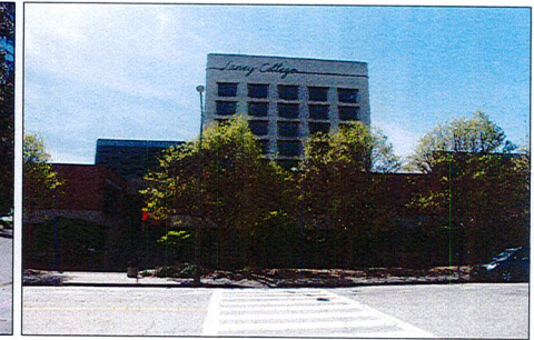
2: Rear (south facade) neighbor, Laney College, from the southwest corner of the building.
