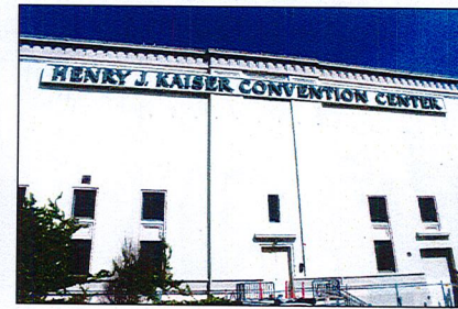
4: View of building rear (south facade) from 10th Street.
