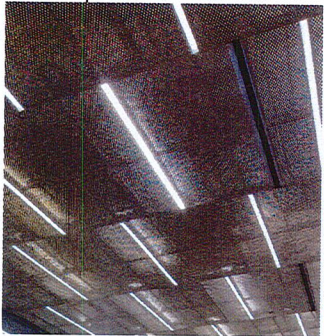
METAL SOFFIT WITH LIGHTS
