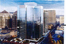
601 CITY CENTER Shorenstein 24 story Under Construction
