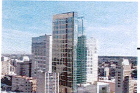
1640 BROADWAY Lennar 380' Under Construction
